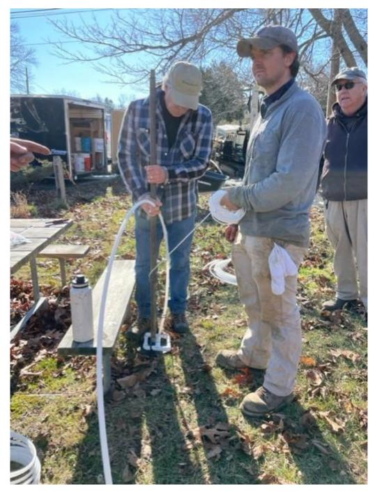
**Figure 3:** Photo of the air injection line before it was lowered into the bottom of the gravel column.
