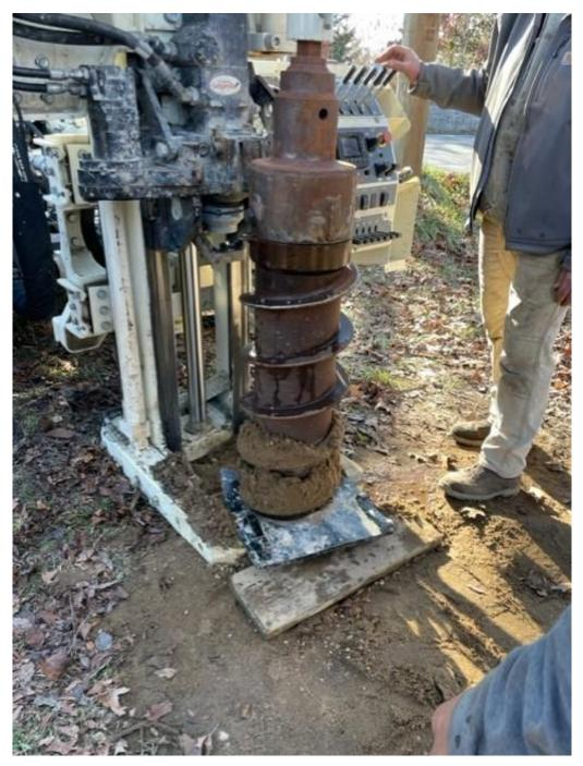
**Figure 2:** Photo of hollow stem auger drilled into the ground to create a ~1ft diameter by 30ft deep column which was then filled with gravel as well as an air injection line and sampling ports.
