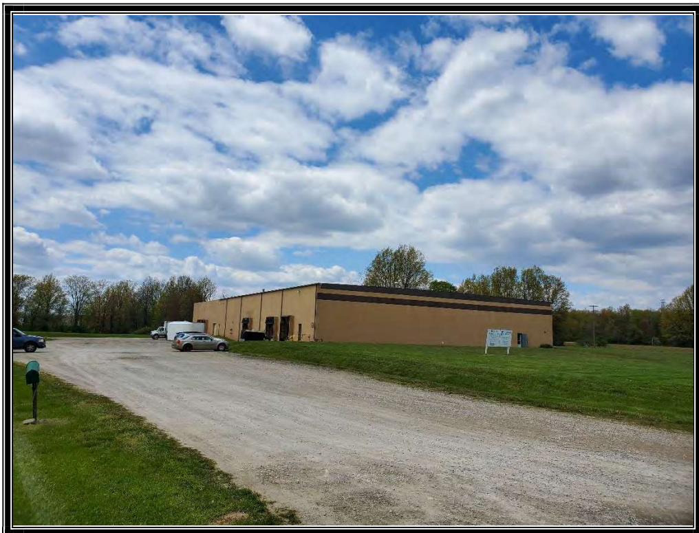
Photo 12: Viewing at K-O-K Products Inc. on the southwest adjoining property.
