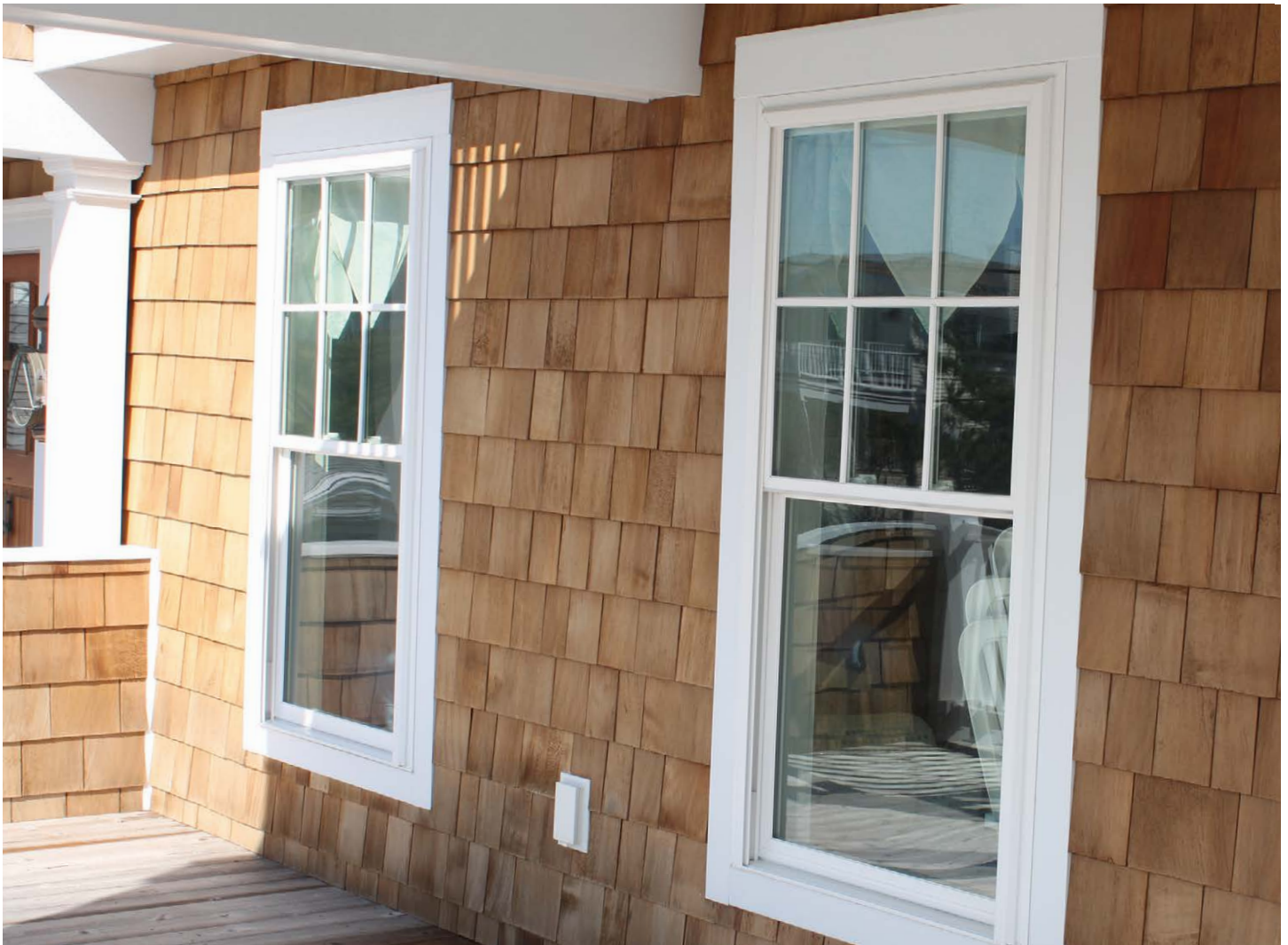
Top: Double-hungs with simulated divided lites, exterior view. Below, right: Close-up exterior view of simulated divided lites
