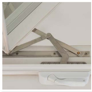
Stainless-steel operator, hinge track, and hinge arm.
