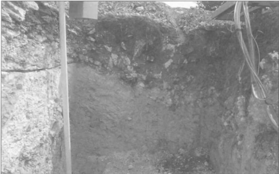
Figure 11.39 This excavation is sloped to allow workers to enter safely.
