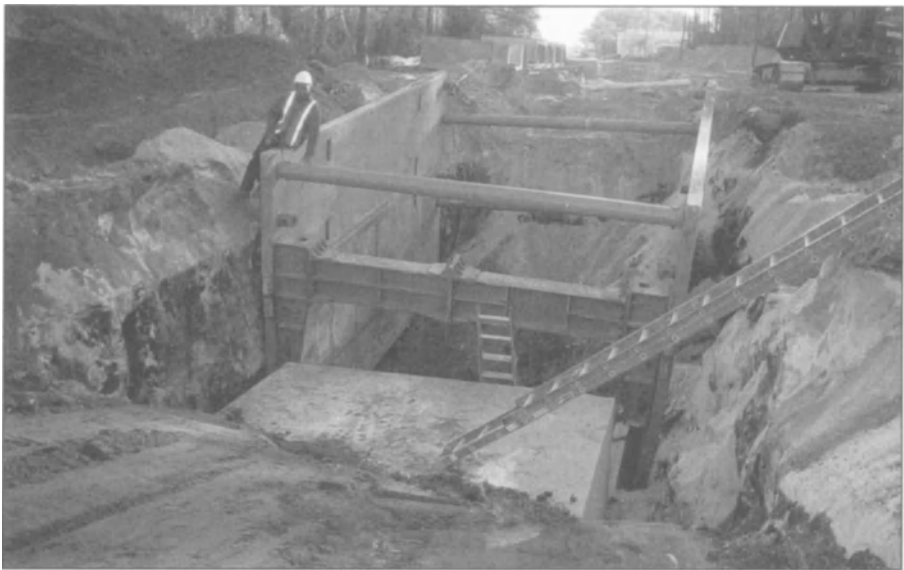
Figure 11.38 This is a trench box. It allows workers to enter the space without fear of collapse of the soil.
