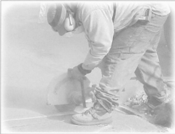
Figure 2.15 This worker, using a concrete cutting saw, is wearing hearing protection in the form of ear muffs to reduce the noise level.
