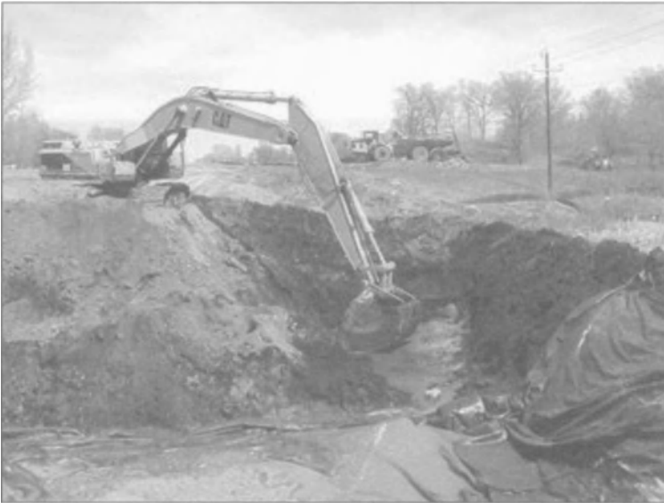
Figure 2.12 This excavation contains petroleum hydrocarbon-contaminated soil which is being removed from a site in Minnesota.
