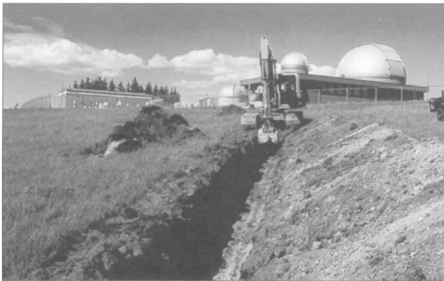
Figure 11.36 This picture depicts a trench being dug to remove chemical contamination.
