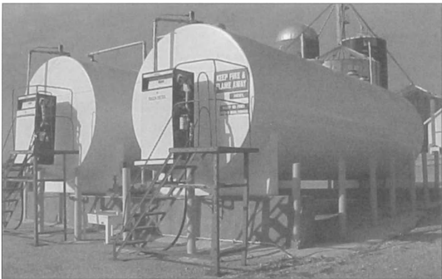
Figure 11.29 This elevated tank has steps that allow workers easy access to it.
