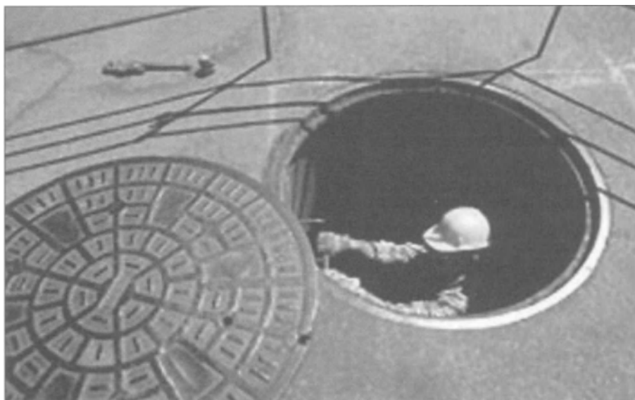
Figure 11.34 A worker is shown inside a manhole (confined space).
