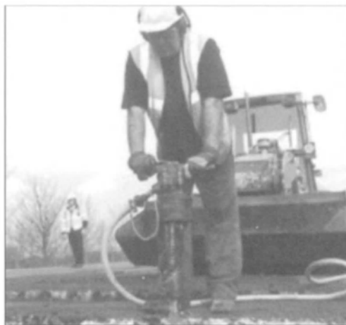
Figure 2.23 This worker is using a jackhammer to remove contaminated concrete. Notice the protective equipment he is wearing.
