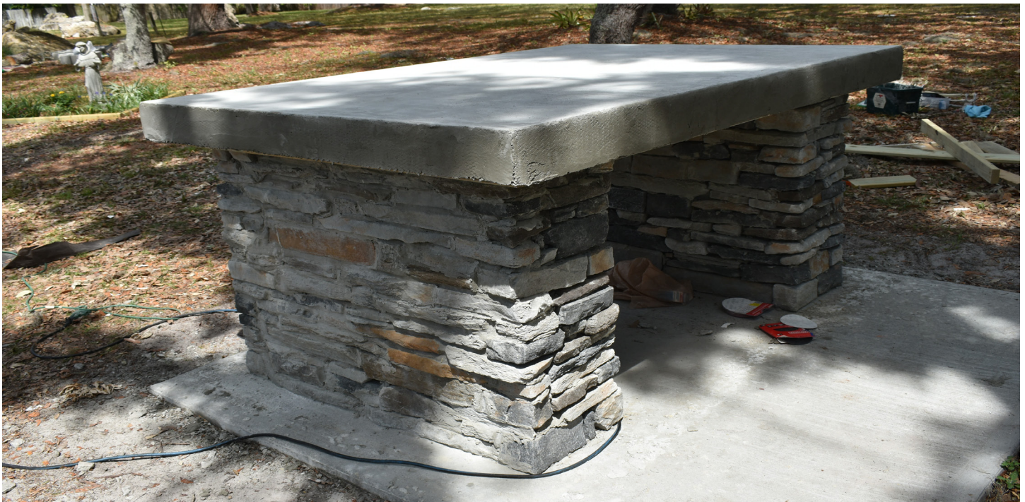
Nearly finished altar sits awaiting decoration around its top edges.
