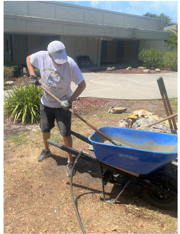
DGK Pete McCabe helps to mix another bag of cement.
