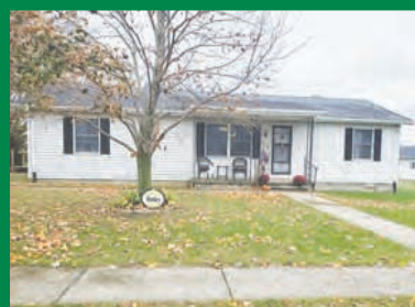
342 N MAIN ST, WEST MANSFIELD - This 3 bedroom ranch home with 2 full baths sits on over 1/2 acre lot across from Memorial Park in West Mansfield. Florida room with large deck for entertaining. Numerous updates inside. Ben Logan School District. Seller is related to agent. Asking $164,900. Call Kimi Ramsey at 937-539-0108.
