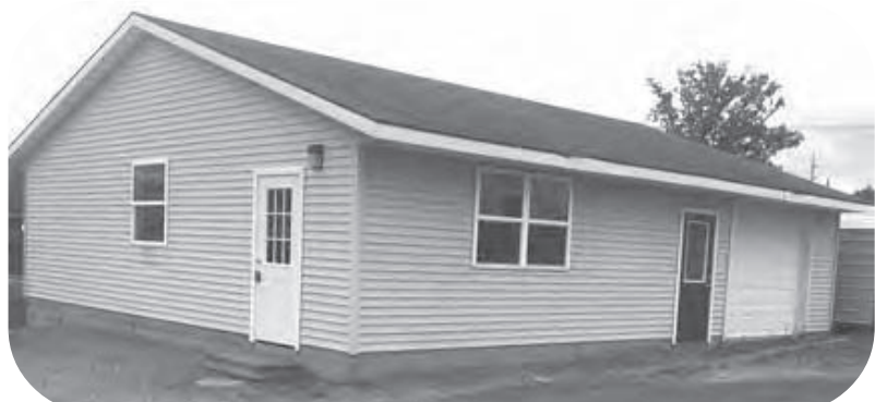
Located at 204 1/2 Lincoln Blvd., Russells Point (far right corner of the Subway/Shopper's Edge parking lot)
