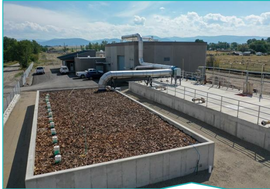
S1 – Augmented Biofiltration
