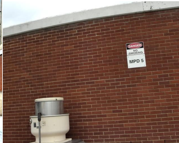
Digester Tank Leak
