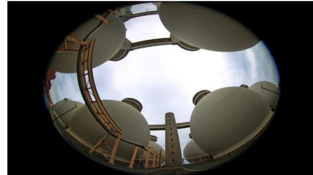
A fish eye view of a wastewater treatment facility in Winthrop, Mass. David L. Ryan/Boston Globe via Getty
