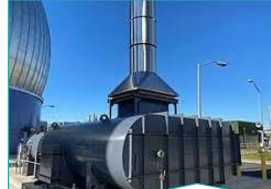
S3 – Regenerative Thermal Oxidizer
