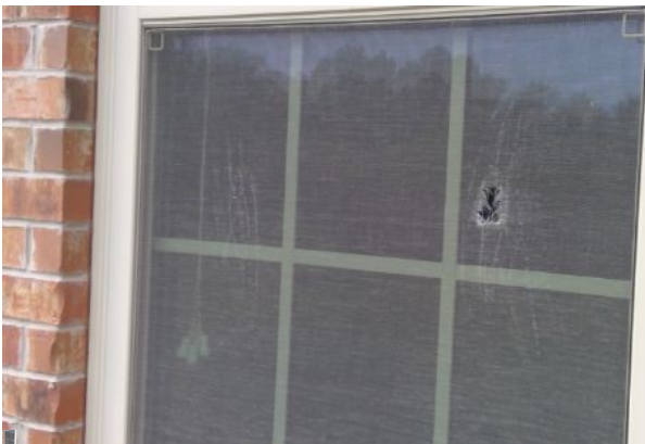
Damaged screens observed.
