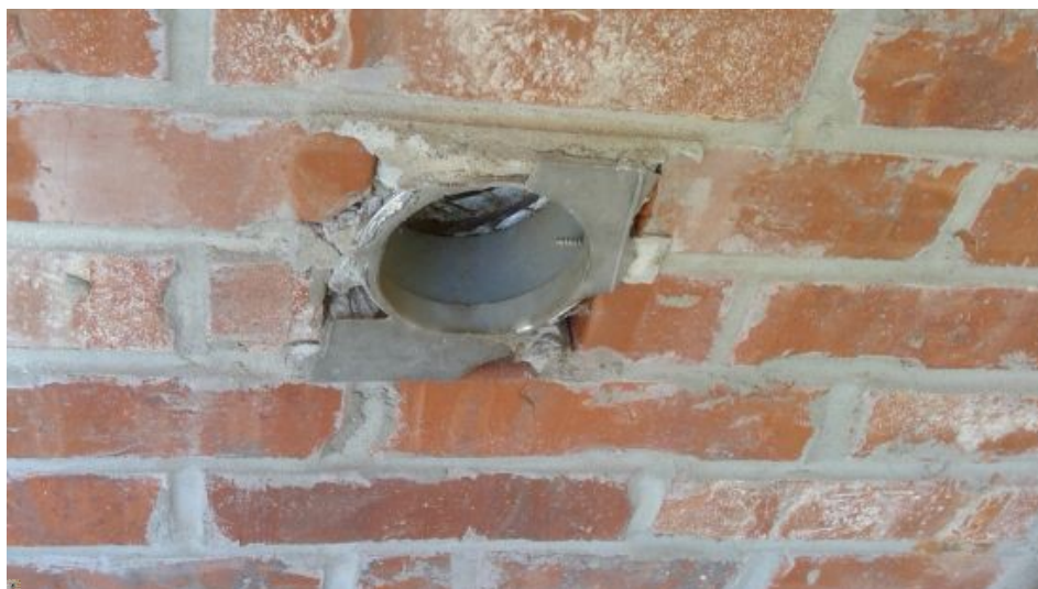
missing exterior cover
