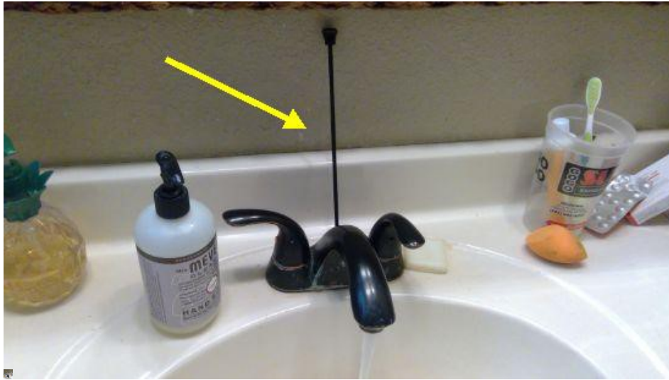
Sink stopper disconnected at master bath
