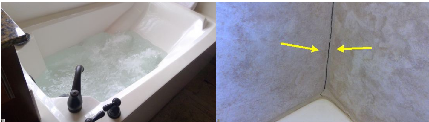
Caulking/grout needed at corners of tub surround in hall bath
