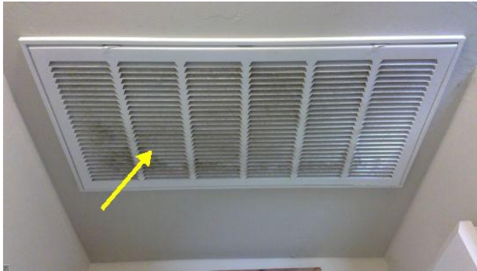
Furnace filter dirty. Needs replacement
