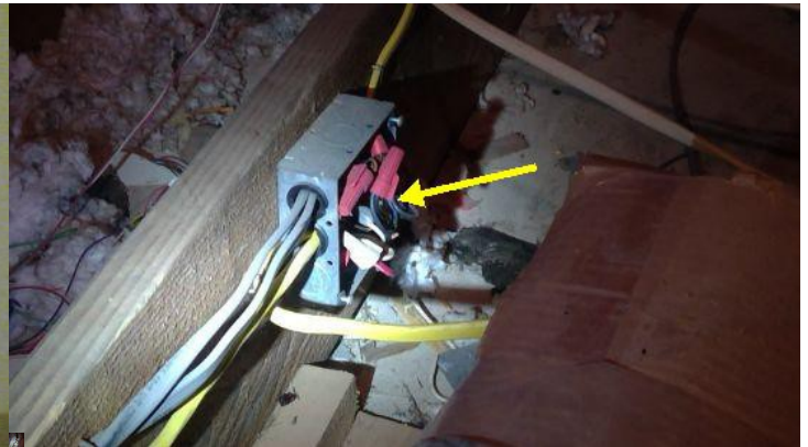
Junction box in attic missing cover plate. Recommend replacing
