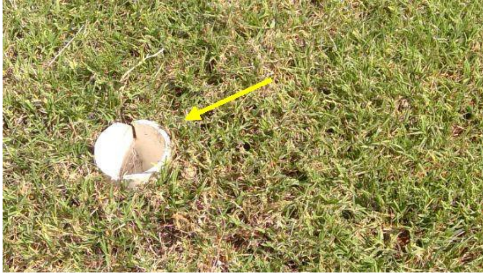
Cleanout cap is missing, recommend replacing
