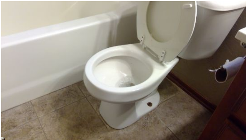
Toilet is loose at the floor in Hall bath, recommend tightening to prevent leak
