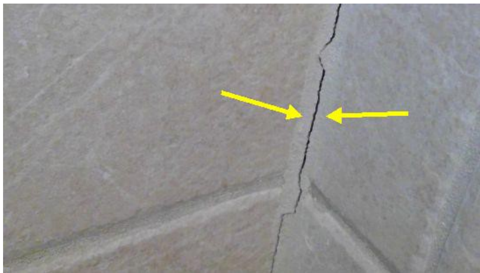
Grout cracking at corners, at & around shower floor in master bath shower. Recommend regrouting or caulking to prevent water damage
