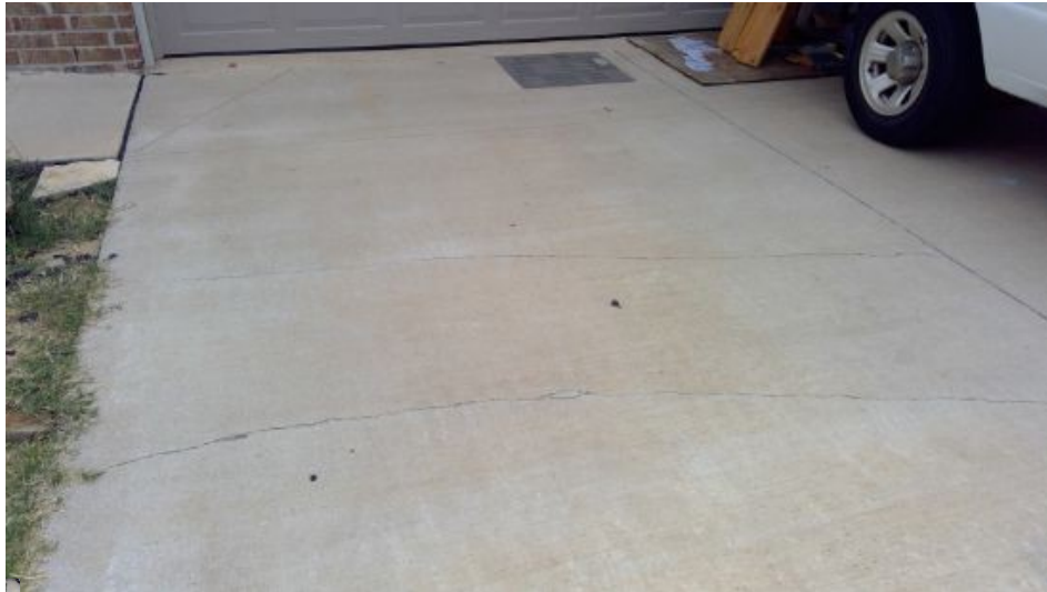
Common cracks, seal as needed.
