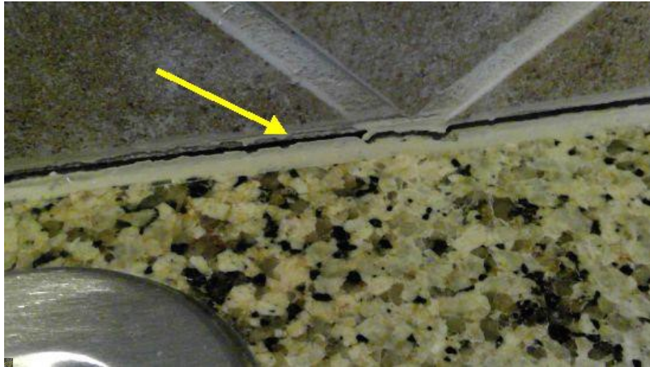
Recommend caulking/grout at Kitchen countertop/backsplash area
