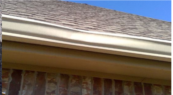
Minor damage noted at gutters. Appears to be functional, repair as needed
