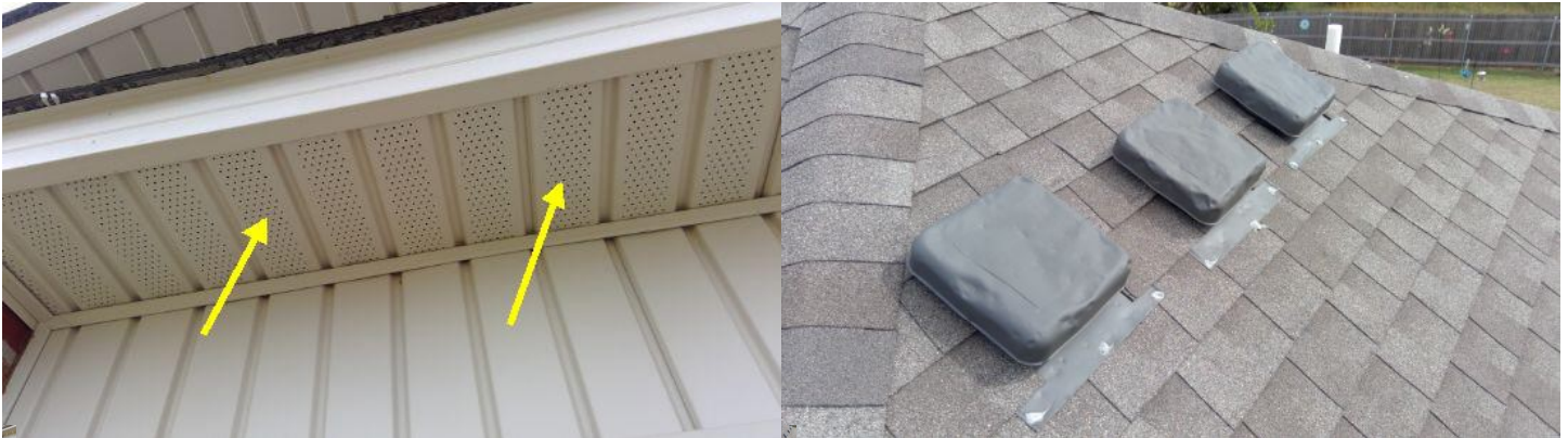
Roof vents are hail damaged, still functional
