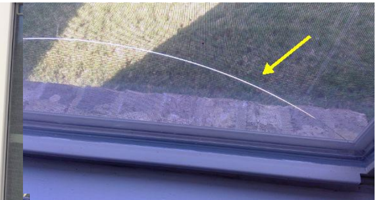
Cracked or broken window glass was observed at north bedroom. Injury could occur. Recommend repair or replacement of the damaged glass.
