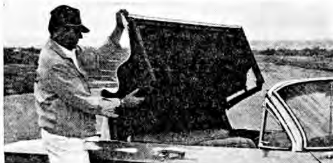
Manually operated top is very easy for one man to handle; it doesn't take any longer to put up or down than an automatic.
