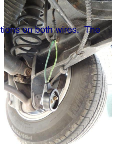
Old connector with wiring exposed
