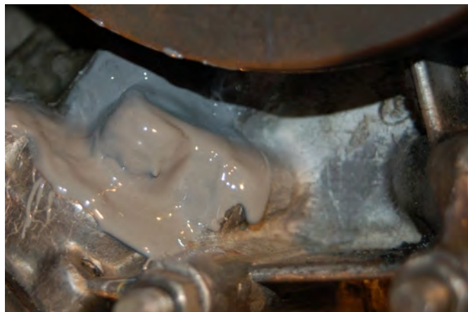
JB Weld applied over shaft bore.
