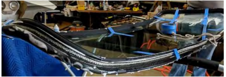
'Body tape' is used to hold the molding in place when you run out of extra hands. Glass, molding and rope is well lubricated and ready to go in the truck
