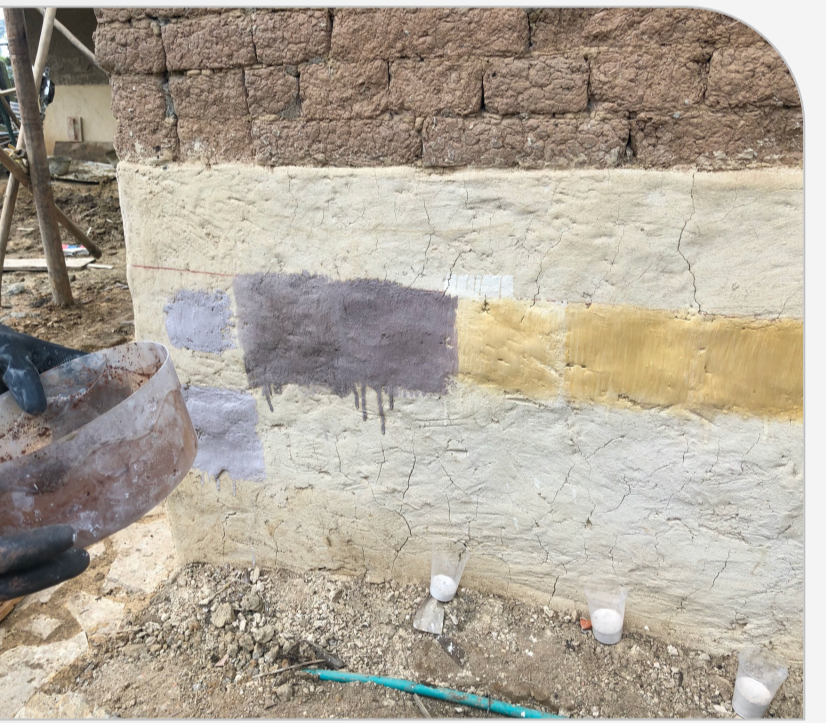
Mineral tinted paint from the site was applied to the facades. 5 type of rocks (minerals) were documented.
