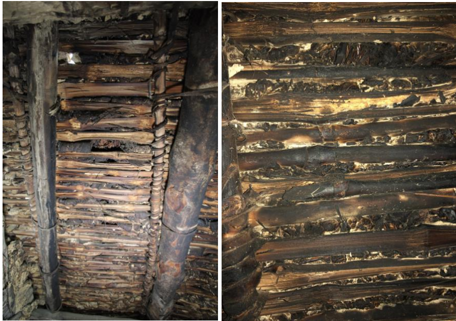
Volume "El Gato". Ceiling made of Andean bamboo, cueron, and clay cured by smoke
