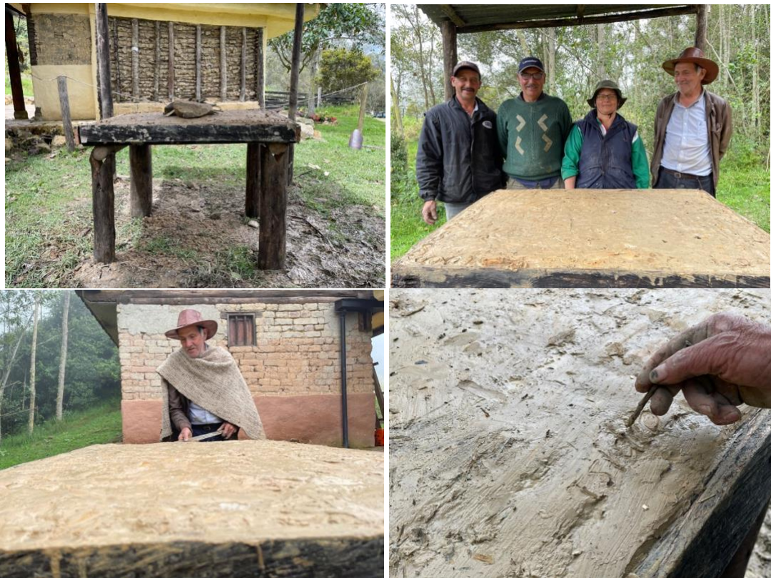
Ancient stone stove rebuilt by local inhabitants. Made of wood, clay and stones.
