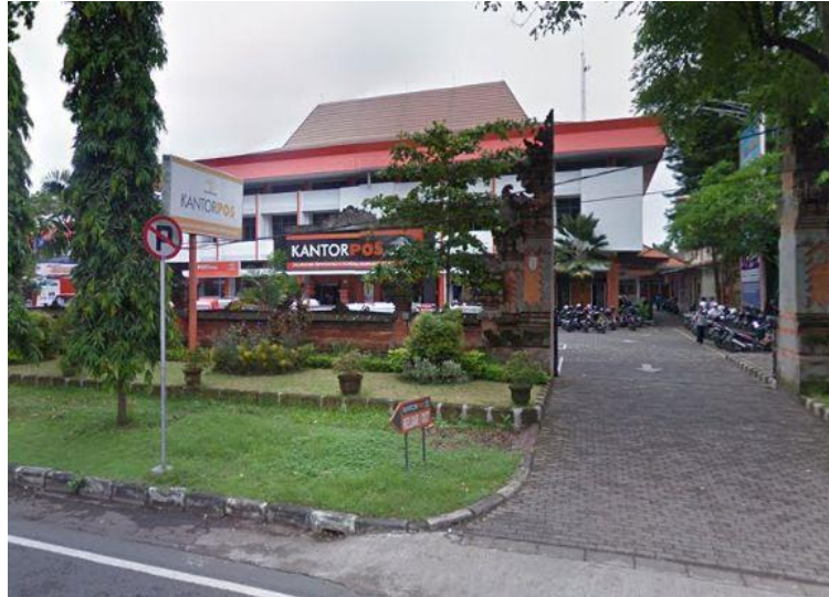
The new Denpasar Post Office building at Jalan Raya Puputan Renon No 37.
