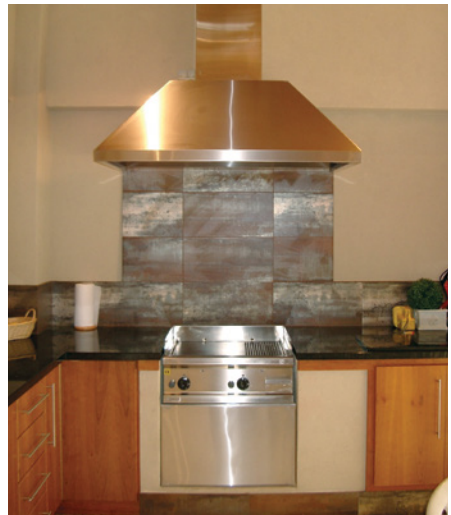
A commercial gas barbecue with mechanical ventilation.
