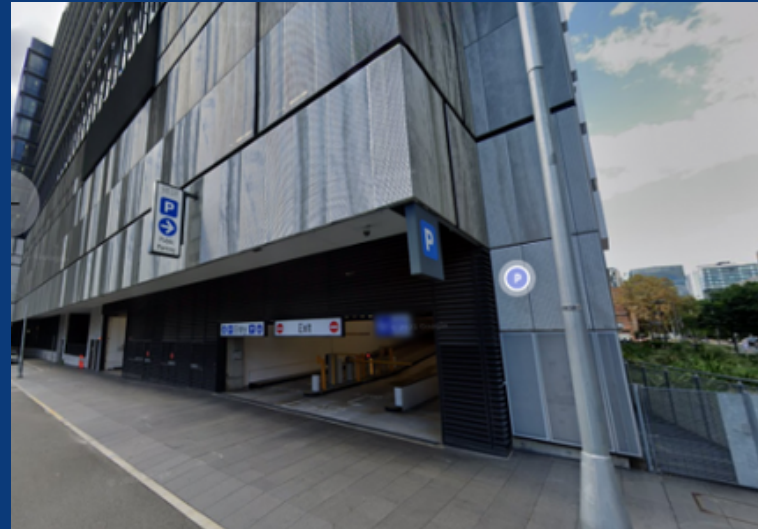
Zollner Cct Parking, Sydney
