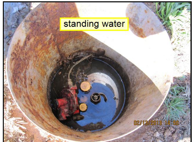
6.4 Item 2(Picture) propane tank valves
