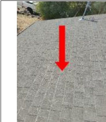
Garage portion showing sun damage of roof
