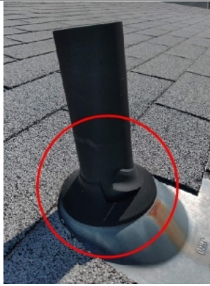
Storm collar needs to be replaced
