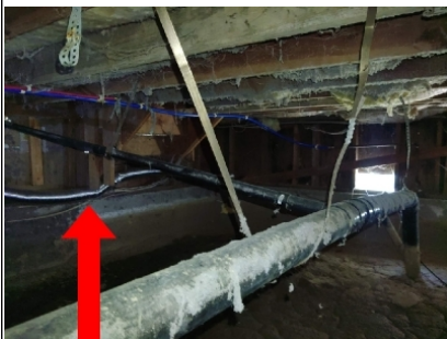
Dryer vent location to exterior wall
