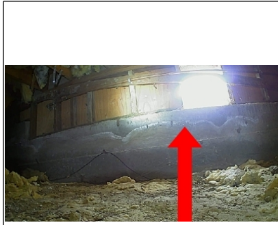
Efflorescence
