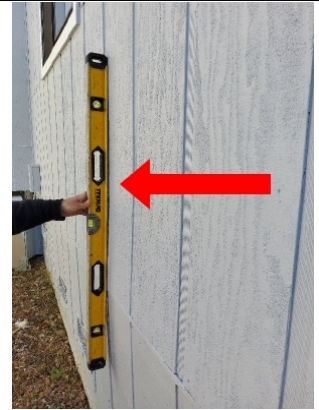
Level is used as a straight edge and shows difference between cripple members and kitchen frame members. This applies the kitchen frame member as the straight edge.
