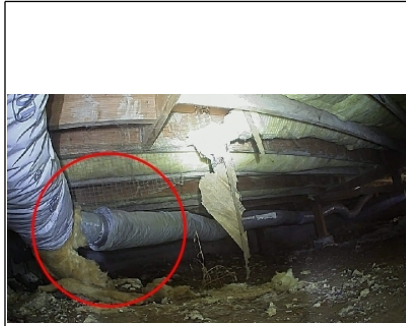
Insulation is evident along with dirt from the ducting in the crawl space.
