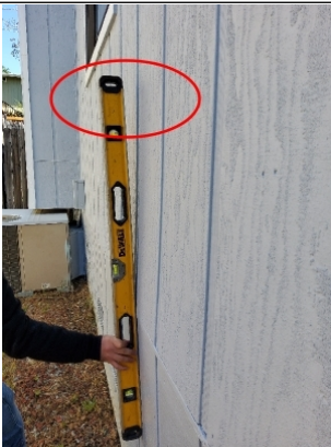
Level is used as a straight edge and shows difference between cripple members and kitchen frame members. This shows the difference between both frame members being out of plumb.
