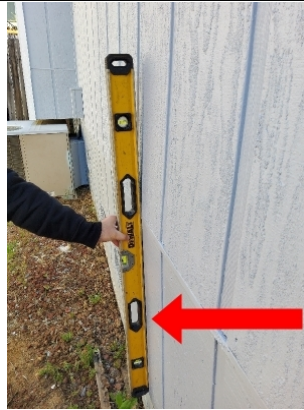
Level is used as a straight edge and shows difference between cripple members and kitchen frame members. This applies the cripple members as the straight edge.
