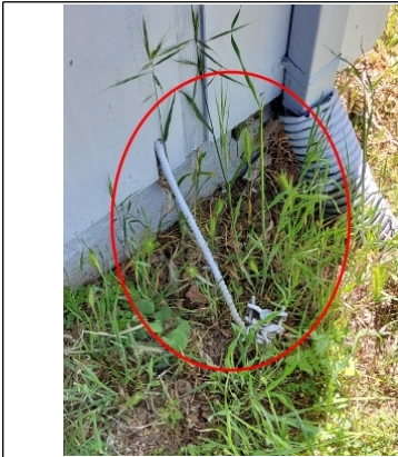
Grounding rod location
