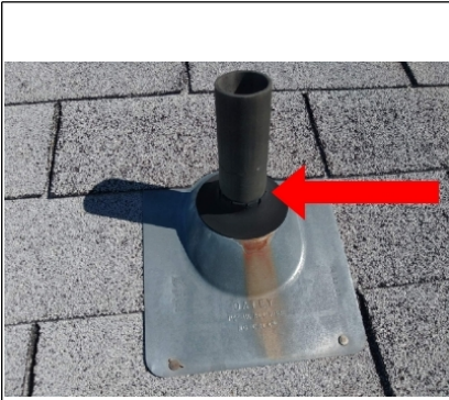
Storm collar needs to be replaced.
