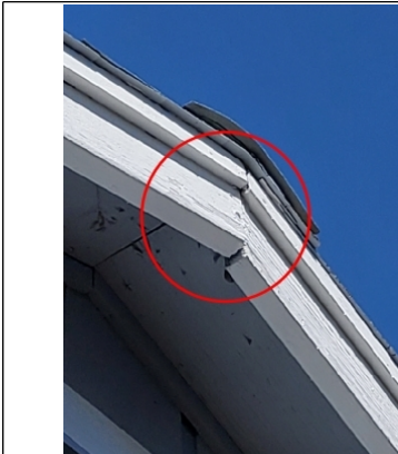
Fascia is twisted from excessive sun exposure and lack of angled screw or nail at the bottom of the fascia member.
