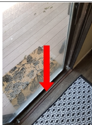
Lubricate door track with WD40
