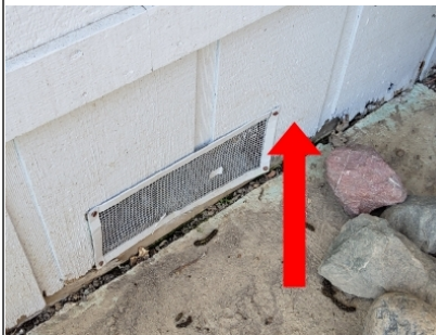
Replace damaged area of siding. would require a section removed with new Z-Bar and new matching T1-11 siding installed.
