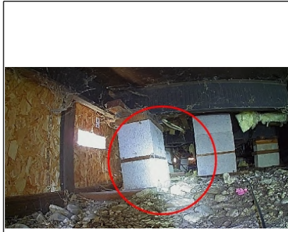
These three pier blocks are leaning significantly.
