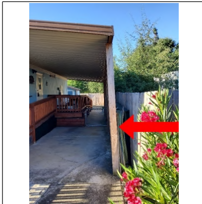
This support post is leaning but is still structurally sound.
