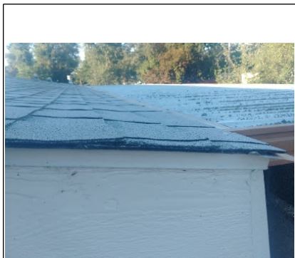
1-layer is properly installed over a starter roll.
