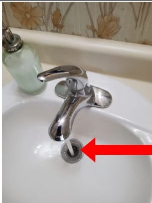
Disconnected drain stop
