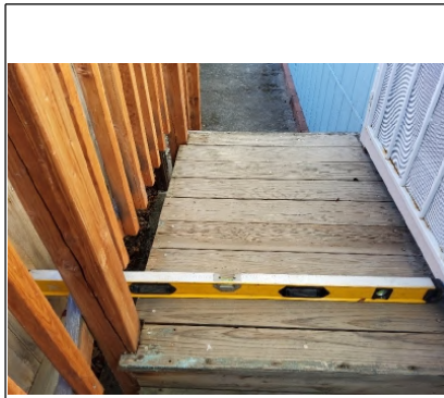
4' level was placed on landing to show it is leaning towards the home.
