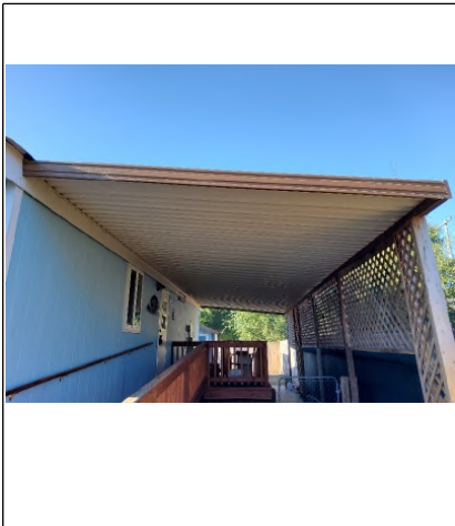
This support post is leaning but is still structurally sound.
