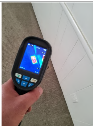
Thermal Imager shows proper "Heat" distribution through vent along with properly sealed ducting at the register.
