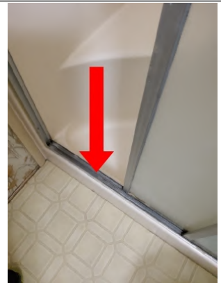
Recommend using WD40 to ease the operation of the shower door.
