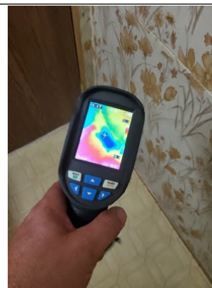
Thermal Imager shows proper "Cool" distribution through vent along with properly sealed ducting at the register.
