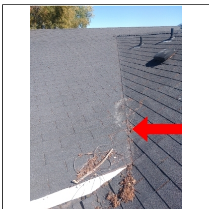
Keep leaf debri away from the valley locations for proper water run off.
