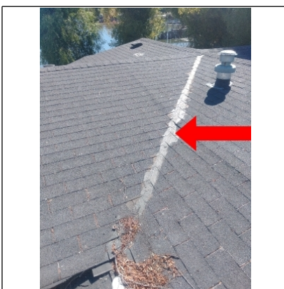
Roof sealant was applied on valley location and for this winter should be resealed with a better sealant product
