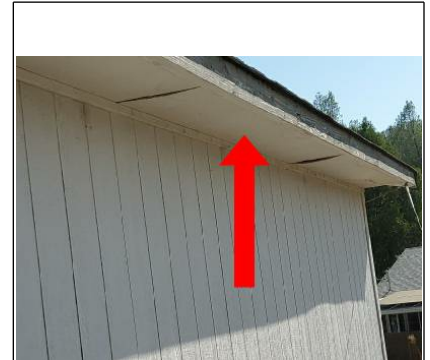
Rotted soffit. Water damage has been evident.
