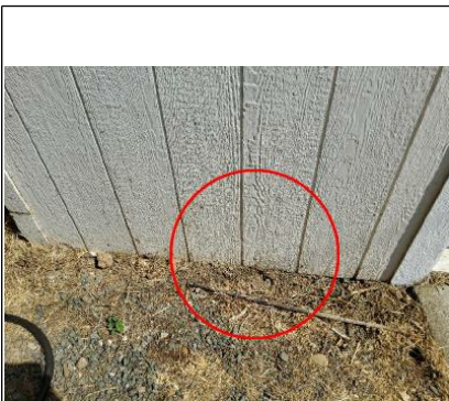
Improper clearance minimum six inches from contact.
