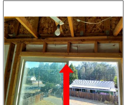
Header needed abice window
