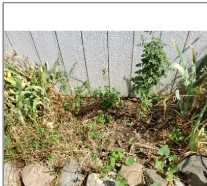
Minimum six inch clearance needed.
