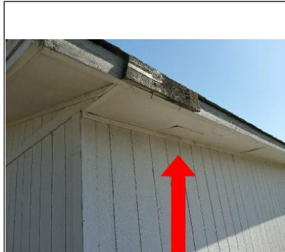
Water damage of possible roof leak. Both outbuilding and house need gutters.
