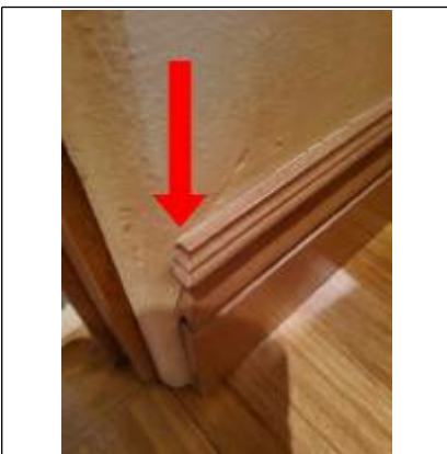
Excellent carpentry on this 45 degree end cut with a micronailer
