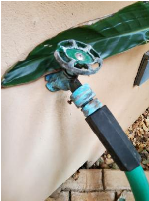
Replace Hose Bib its Leaking (Location front porch)
