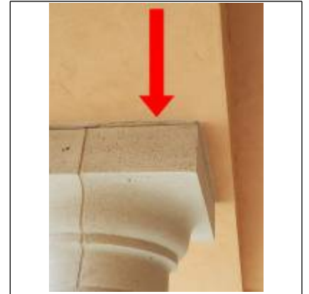
Crack can be regouted
