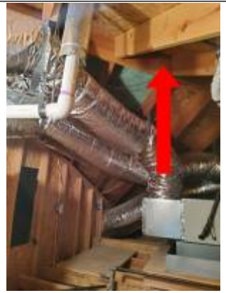
Cut and Stack rafter to ridge
