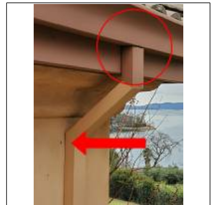
Missing Bracket for downspout and can be refasted to gutter
