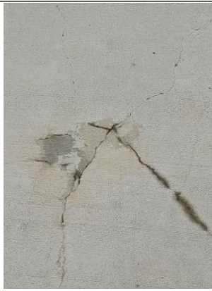
Non-Piercing Settling Crack
