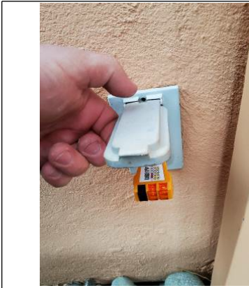
Proper GFCI Connection
