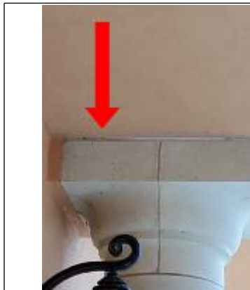
(Right Column) Crack can be regouted
