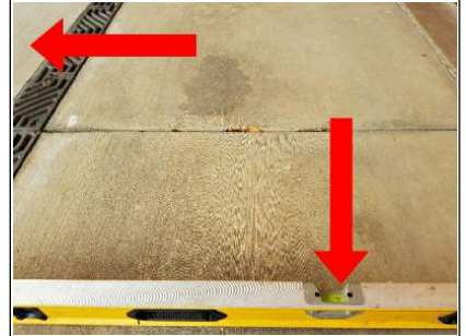
This shows proper fall to the drain tile. This is another example of attention to detail, the pitch of (Left Arrow) driveway is pretty shallow that the concrete contractor could have made this flat because the drain tile would still collect water run-off.
