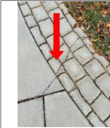
Standard settling crack did not pierce through less than 1/4 of inch wide.
