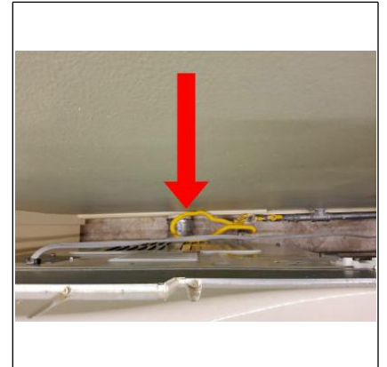
Dryer Vented to wall properly with proper material
