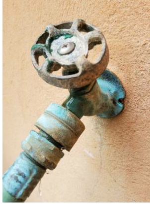
Replace Hose Bib its Leaking (location between right porch and garage )
