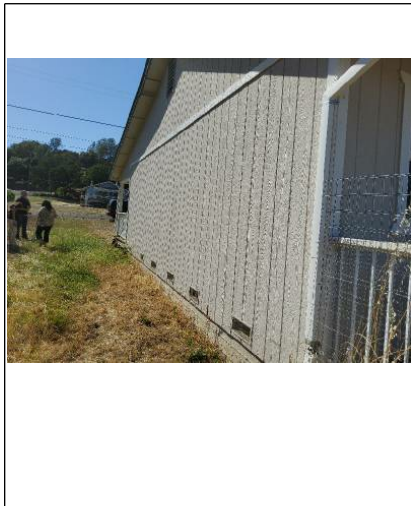
Siding below six inches. must have minimum six inches of clearance of ground.
