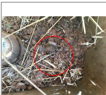
Leak has been found
