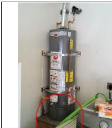
No over flow pan. This is an electrical hazard
