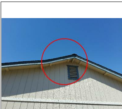
Top Fascia piece needs to be replaced
