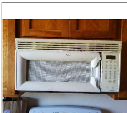
Must replace microwave. Unacceptable
