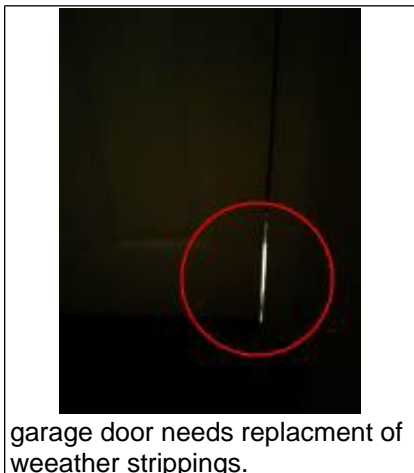
Garage door needs new weather stripping
