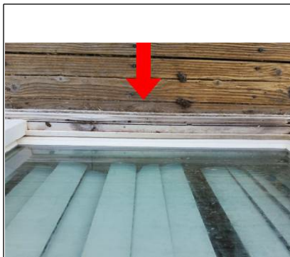
Bottom sill damage on back patio door
