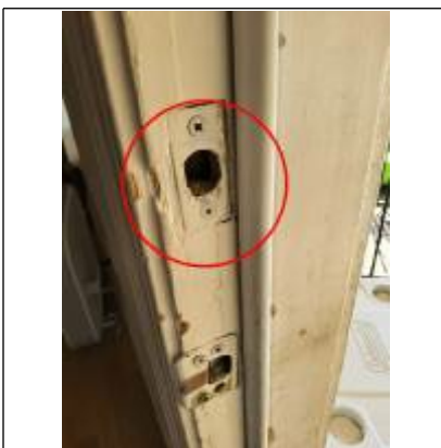
Not properly installed as door has issue closing
