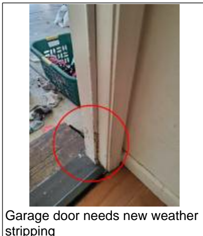
garage door needs replacment of weeather strippings.
