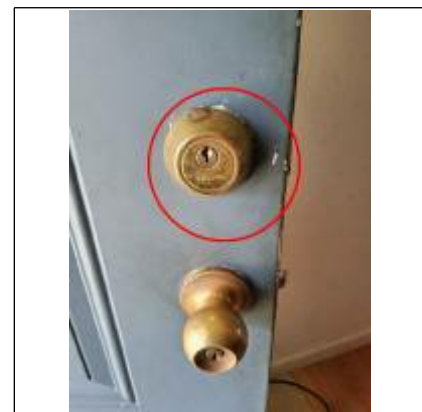
Not installed correctly.
