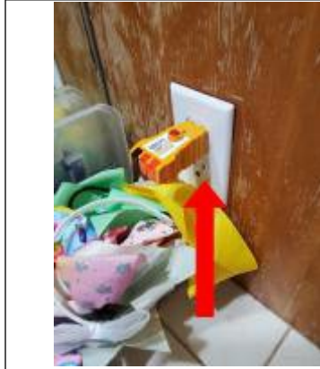
Not proper GFCI in Master Bathroom
