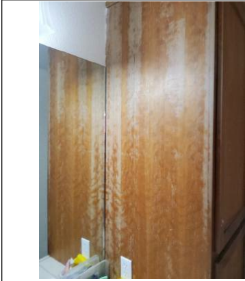
Cabinet is worn
