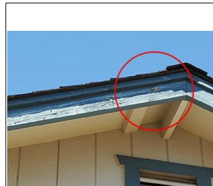
Wood damage from sun needs to be replaced
