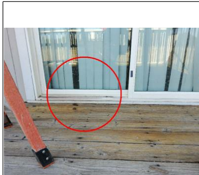
Some damage on bottom sill. also need to rechalk around the trim on inside butting the frame of slider.
