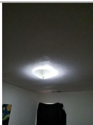
Recommend Ceiling fan
