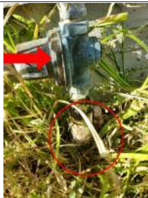
slow leak is also noticed at the connection. Furthermore, recommend replacing water pressure reducer as corrosion is shown this is the source of the issue with low water pressure in the house.
