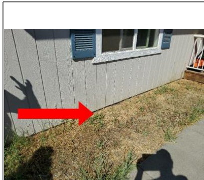
Siding below six inches. must have minimum six inches of clearance of ground.
