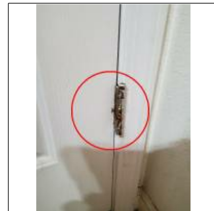
Rust on hinges in bathroom need to be replaced
