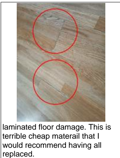
More damage on flooring
