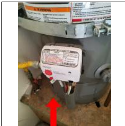
A pan is needed below all hot water heaters
