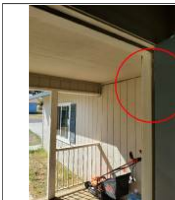
Replace weather strippings on front door.
