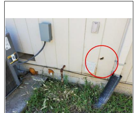
Massive hole in the wall needs to be chalked or spray insulation
