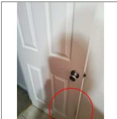
Damage on door
