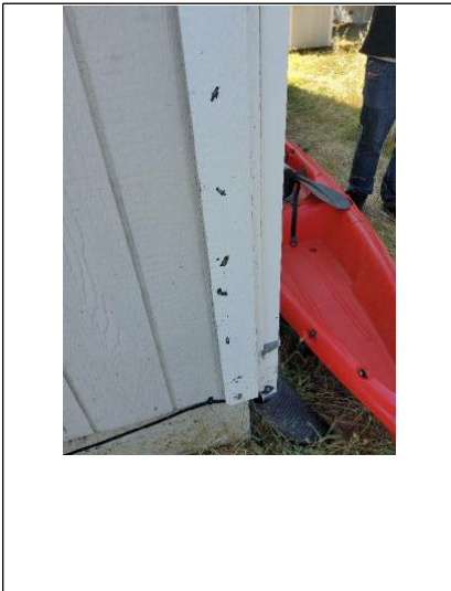
Some damage on bottom sill. also need to rechalk around the trim on inside butting the frame of slider.
