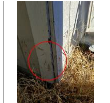
Rot damage, needs to be replaced
