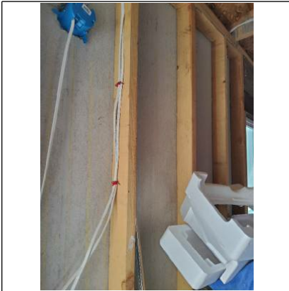
No shear! this is the garage where you can also see no vapor barrier.
