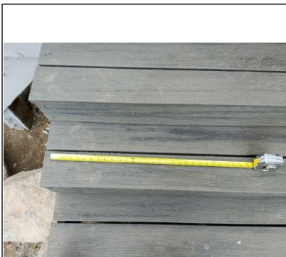
Steps on back deck need to be 16 on center risers. This is two feet which would work for standard 2x6 wood decking but not Trex.
