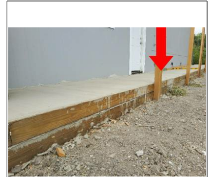
These foundation forms should be pulled as the general claimed he left them there for fencing? so he would go horizontal with the planking? This does not make any sense. the 2x4 horizontal piece would have been in between the posts so there is no point. Also this looks terrible! u can see this from the road.
