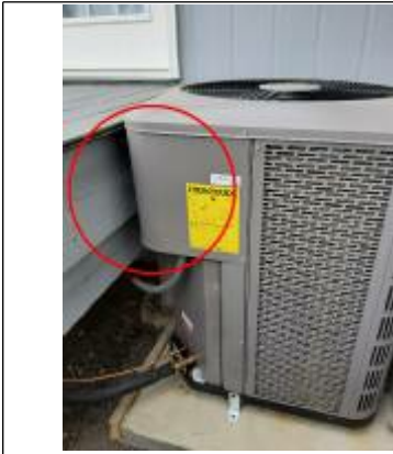
How can this unit be accessed, let alone see what the Serial and Manufacture number is for ordering parts?
