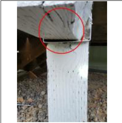
girder is not sitting directly on post mounting hardware / strong tie
