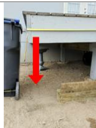
no support for rim especially if this is not tied into the house rim.
