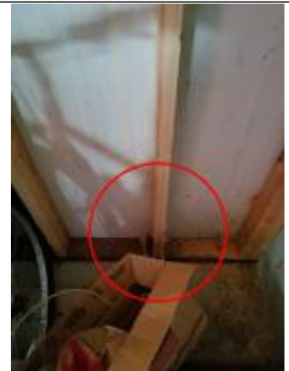
Interior side of wall no block support or shear for illegal paf
