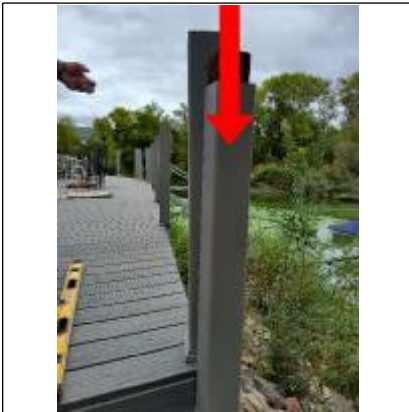
Extremely out of level look at the post compared next to it.
