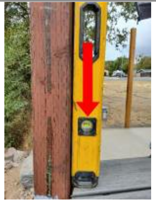
This is almost an inch out of level and this was considered not the worst post.
