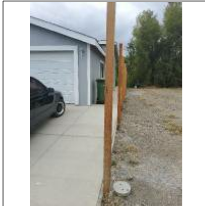
These are doug fur posts and should not be installed in dirt. also this contractor clearly did not run a string line for these posts.
