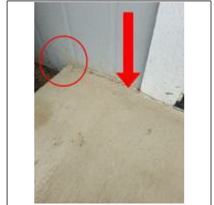
Refer to circle on this one... that its 4 inches atleast of concrete up against the hardie plank with no added support behind the siding!
