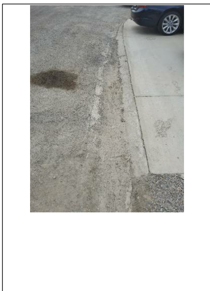
Foundation forms were not setup properly or string lined with stakes to keep a straight line.
