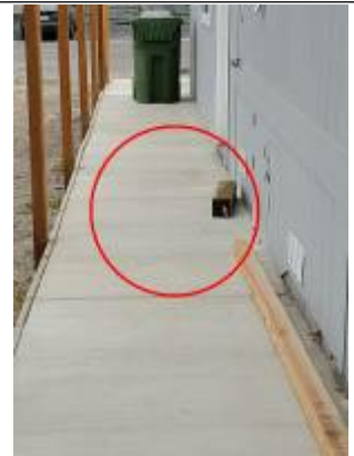
This is guaranteed to be a puddle area where water will just sit.
