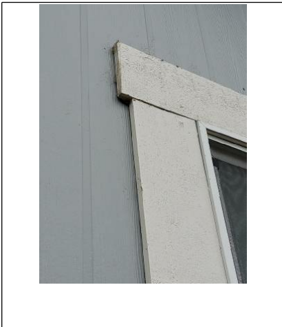
Wood trim should not be touching concrete
