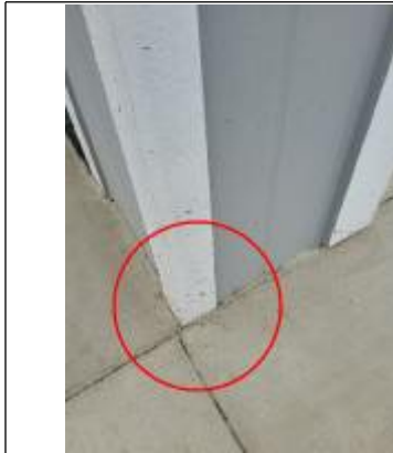
Wood trim should not be touching concrete this will rot.
