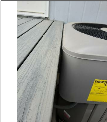
Model serial number all covered which makes service merely impossible along with inability to access unit.
