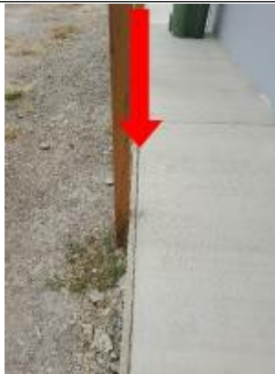
If you see in person and view this arrow u will see how far out this slab is as well as the posts.
