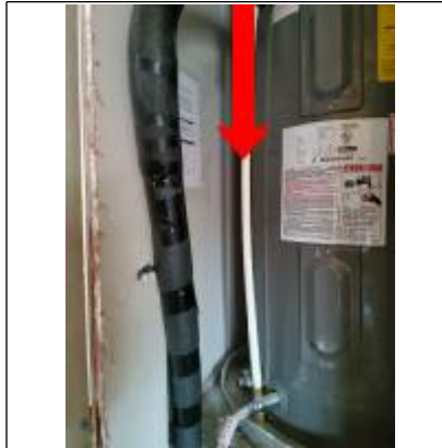
Relief valve is suppose to be copper.
