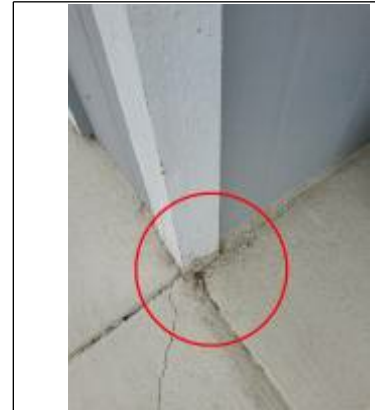
Wood trim is imbedded in the concrete, unacceptable!
