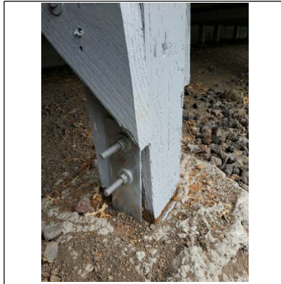
Again this needs to be lags not bolt and washers.
