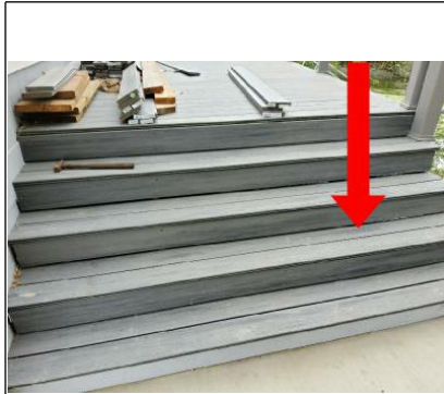
Same goes for this back deck. Deck treads need to be taken off and more stair stringers need to be installed for a 16 on center spacing.
