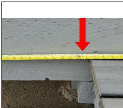
Cantilever past four feet not code.
