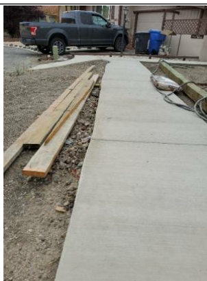
Was there ever a drain tile installed? after the house was put in place? Especially got gutter downspouts?
