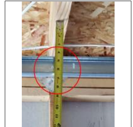
Left side 4.5 inches from truss to top of garage door track.
