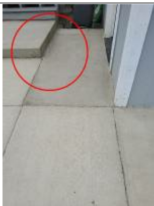
Terrible botch finish concrete job
