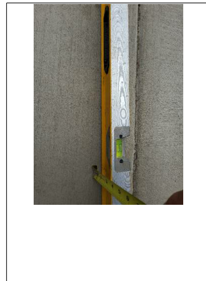
This is fall towards the house not away. This is unacceptable, no concrete person should ever consider this ethical to have water fall to the house.
