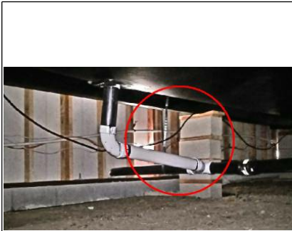
Metal straps should not be used on ABS or PVC
