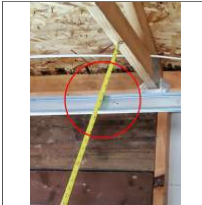
Right side 7 inches from truss to top of garage door track.
