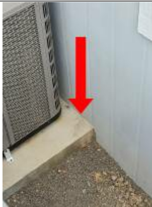
Concrete pad poured refer to next photo after to show otherside of wall.
