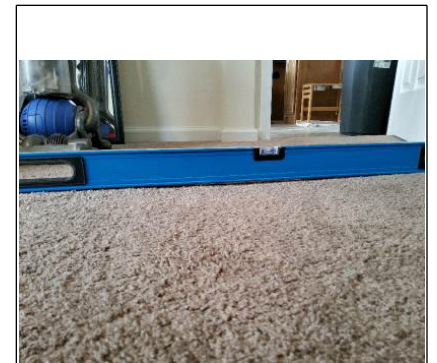
1/4 inch dip where the units meet.
