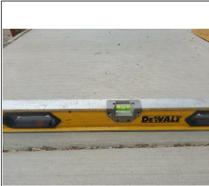
Not proper fall in front of crawl hole.
