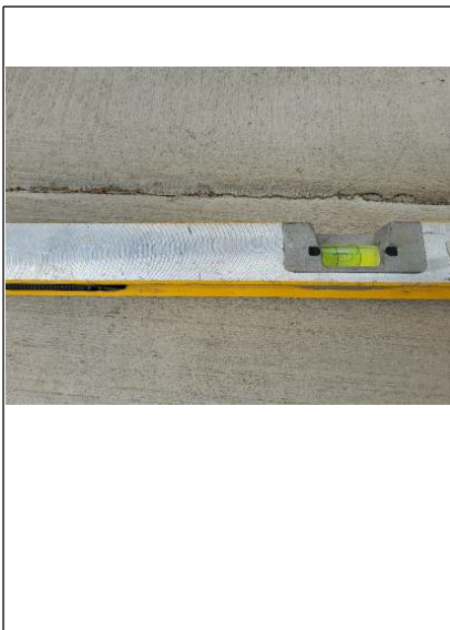
over an 1 1/2 inch fall at four feet towards the houuse. This will erode the hardie lap siding especially since the skirt board has no sheer.
