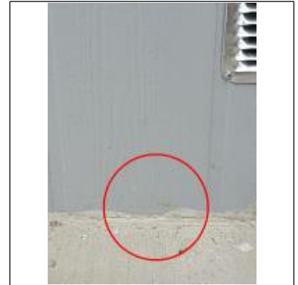
Concrete butting the siding this is a terrible HACK JOB!
