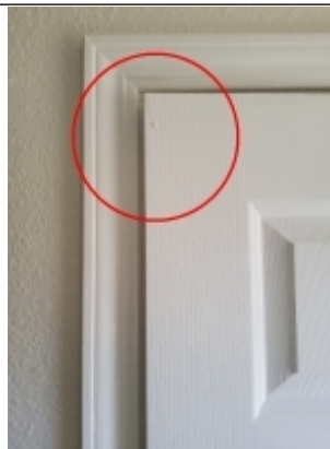
Door rubbing Jamb (Refer to Next slide for solutions)
