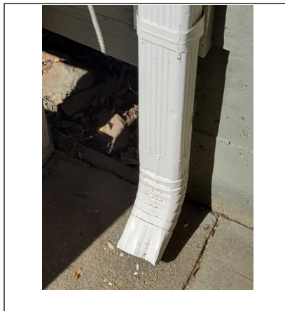
Missing Elbow
