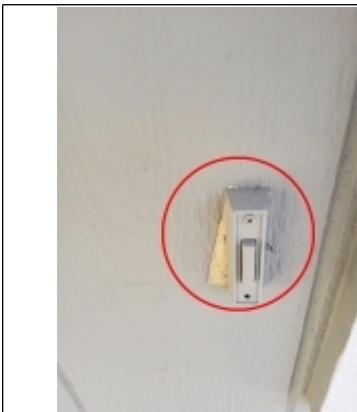
Refasten door bell and touch up paint
