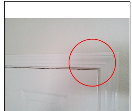
Door rubbing (Refer to Next picture for solution)
