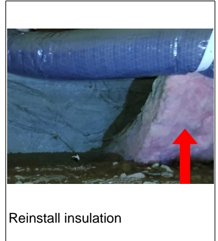
Various insulation batts are not between joist members.
