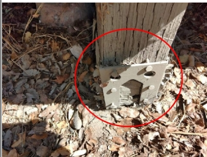
Refasten Joist nails in column
