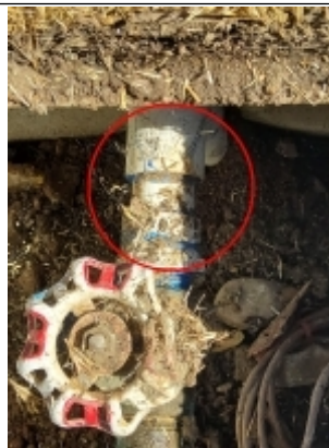
Slight leak on PVC Connection
