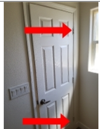
Replace existing center screw just one in each jamb. Predrill and match the head at local lumber store, install a 3" screw after predrilling, this will tighten the jamb to the trimmer.
