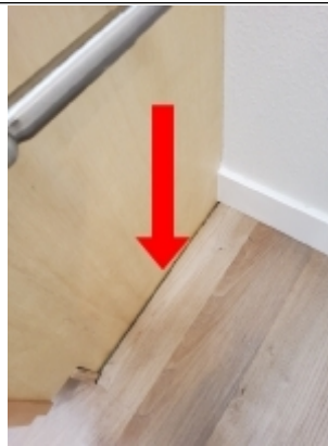
Missing trim member. Recommend installing quarter round or baseboard.
