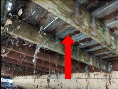
Slight Moisture Damage underneath planking members.
