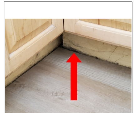
Quarter Round will have to be applied after installing new toe kick as the space from hardwood floor to cabinet is too far to fur-out.
