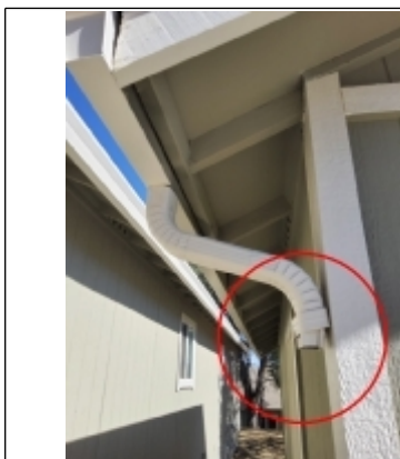
Missing Downspout
