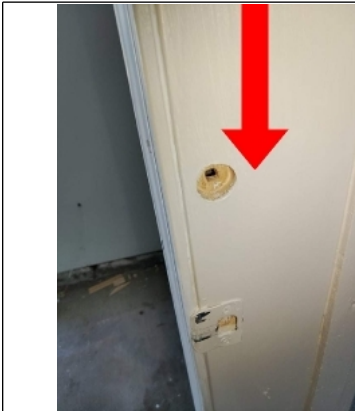
Missing Jamb Stop and Weatherstripping
