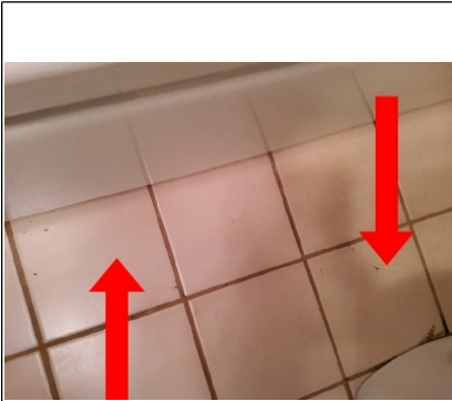
Slightly cracked tiles
