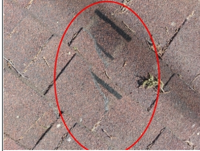
Damaged shingles
