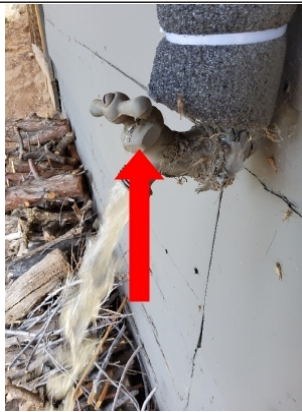
Replace leaking hose bib.
