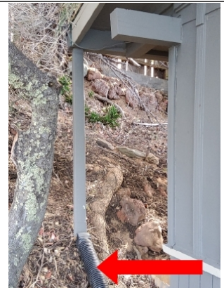
Downspout has proper drain tile extension to keep run-off away from perimeter foundation wall.
