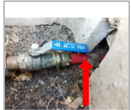
Water entry material is PEX Plastic
