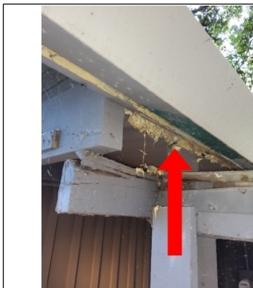
Spray foam was applied to reduce chances of insect intrusion.
