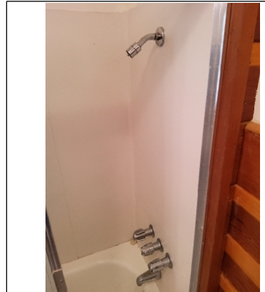
Replace diverter valve
