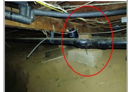
Girder member and footing are the reason for the slope.
