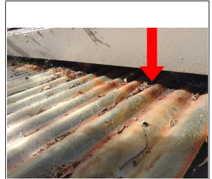
Gutters are leaking which explains the rust on porch cover.
