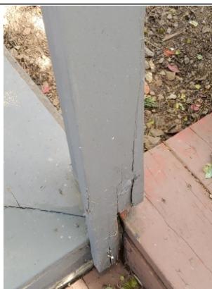
Slight moisture damage is evident on 2x4 wood member.
