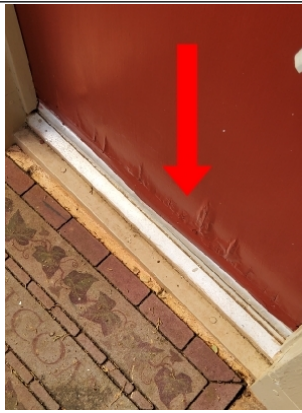
Damaged door slab. Recommend having exterior door replaced.
