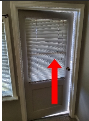
Recommend replacing interior door with an actual exterior door.
