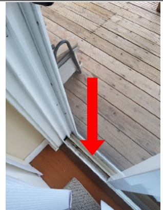
Lubricate sliding door track with WD40
