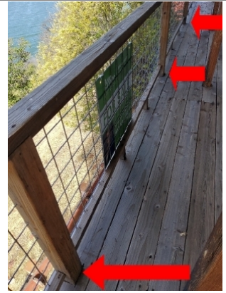
Loose posts. Recommend installing Simpson Strong-Tie L galvanized steel angle strap. (Refer to next slide for item)
