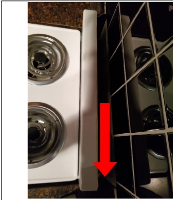
Missing anti tip bracket
