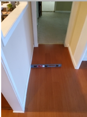
2' Level shows slope on floor.
