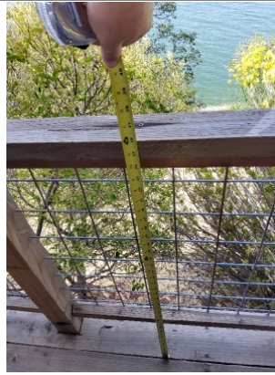
Railing meets code requirements for when it was built 36"
