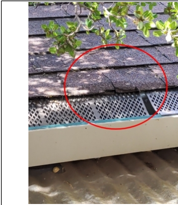
Damaged Shingles
