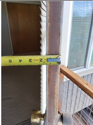
The current exterior door is not an exterior door. This is an interior door it is 1-3/8" while exterior doors are 1-3/4".
