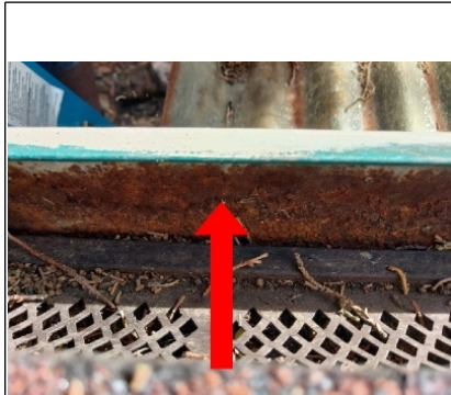
Gutter is improperly sloped to downspout. (Arrow points to the center of the bubble that shows improper pitch to downspout)
