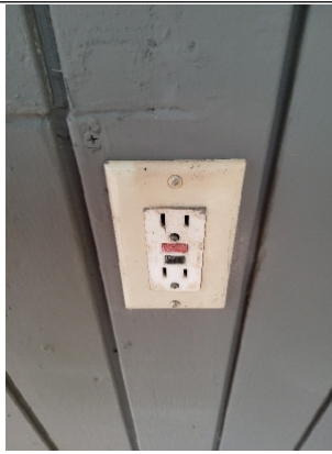
Electrical outlet is missing proper exterior outlet cover.
