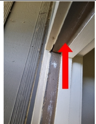
Install weatherstripping
