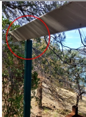
Improper pitch gutter to downspout referenced to prior slide.
