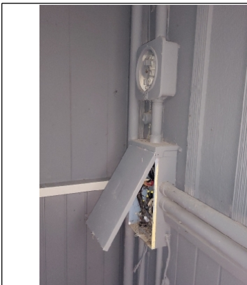
Disconnected (Original Panel Box)
