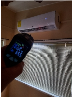
Thermal Reader shows proper AC distribution
