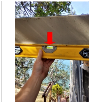
Gutter is improperly sloped to downspout. (Arrow points to the center of the bubble that shows improper pitch to downspout)
