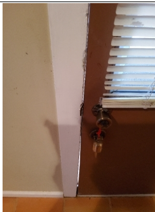
Damaged door slab. Recommend having exterior door replaced.
