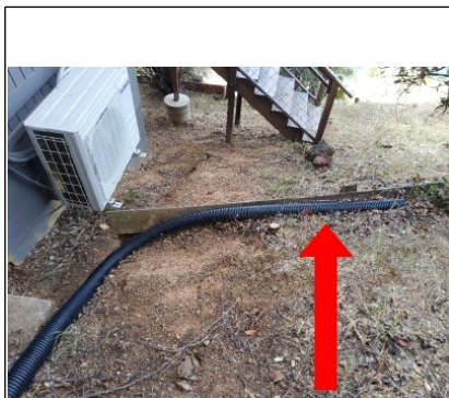
Corrugated drain tile is properly diverting water run-off away from the perimeter structure.
