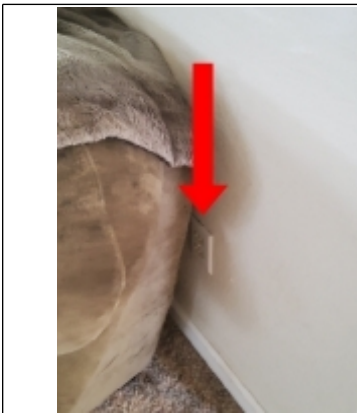
Tighten outlet cover
