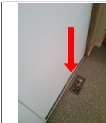
Slightly bent closet door
