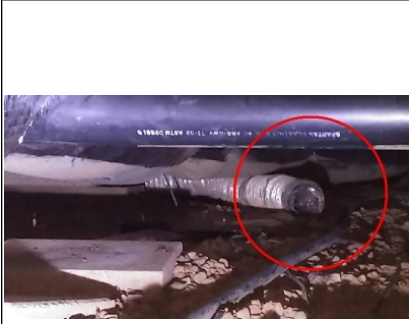
Disconnected Dryer Vent
