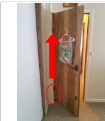
Door stop needed. Making bottom hinge pull away
