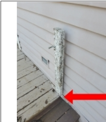
For now before removing deck. Change out bottom bracket and replace with straight galvanized bracket to tie in rim board.
