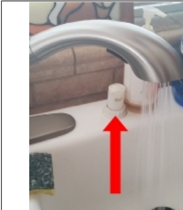
Missing Dishwasher Air Gap Cover
