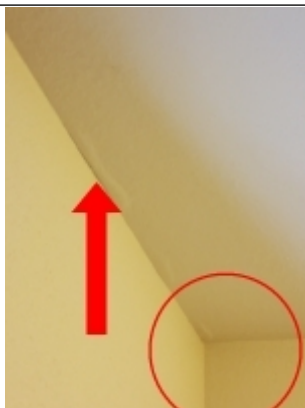
Bubble on tape joint not a leak
