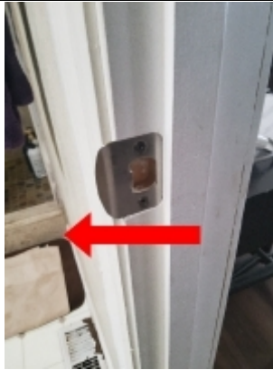
Move strike plate to left to properly latch door. Make sure you predrill new holes prior.
