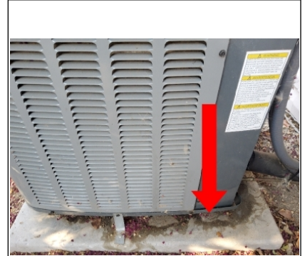
Perfectly normal this is defrost. The hotter the exterior tempature the most defrost will be evident this is a new unit that is less then 4 years old.
