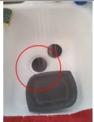
Grinding sound most likely debri trapped in chamber
