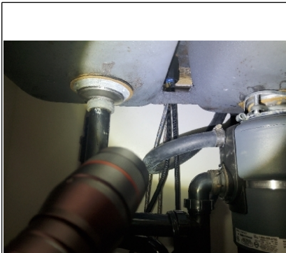
Missing Dishwasher Air Gap Cover
