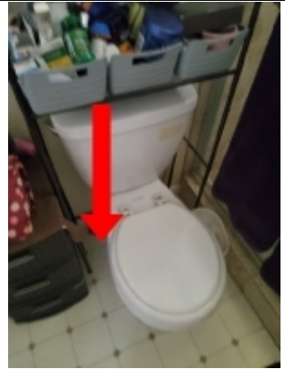
Toilet is a hair loose on the base can easily be tightened
