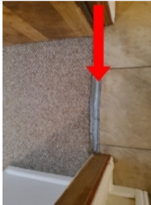
Install mold cap between tile and carpet
