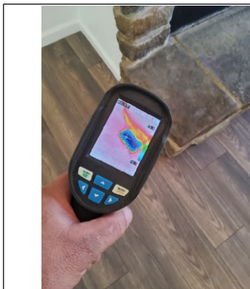
Thermal Imager shows proper "Cool" distribution through vent along with properly sealed ducting at the register.
