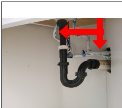
Recommend removing all painters tape from flex supply lines.
