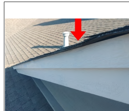
1-Layer of asphalt shingles are installed over a starter roll.
