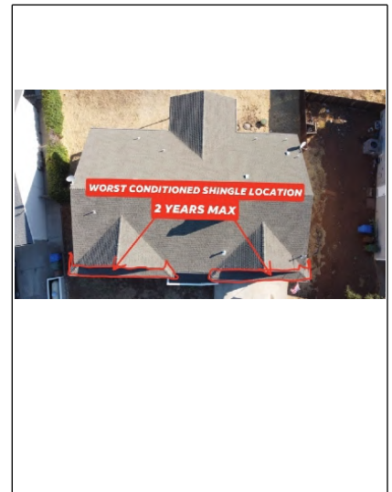
Accurate representation condition of the roof shingles with reference to prior drone diagram. (3 Years of Life Left)
