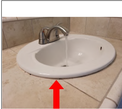
Recommend using Custom Building Products Polyblend Haystack Silicone Acrylic Tile Caulk to properly seal between tiles.
