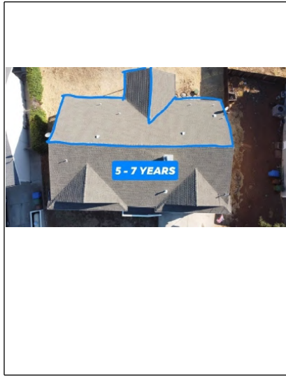
Accurate representation condition of the roof shingles with reference to prior drone diagram. (3 Years of Life Left)
