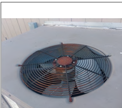
Rust is evident on grill cover. Recommend having replaced by a Licensed HVAC Contractor.
