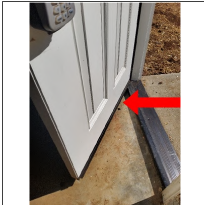
Recommend replacing existing door sweep as the door does not properly swing without scratching threshold.
