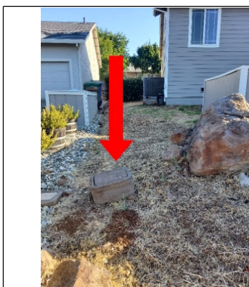
Water meter location
