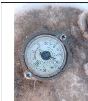
Propane tank is 77 percent full during time of inspection.
