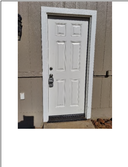
Recommend replacing existing door sweep as the door does not properly swing without scratching threshold.
