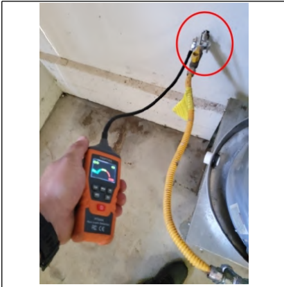
No leaks were detected on shut off valve.
