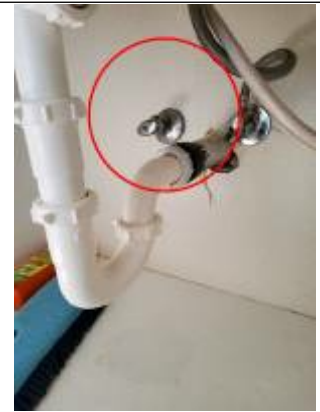
Disconnected flex line recommended adding new flex line to sink
