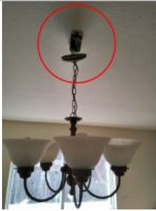
Dining light needs to be reattached and adjusted.
