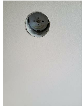
Missing light fixtures in two openings.
