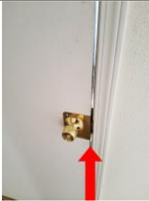
Replace the weather stripping with a thicker weather stripping to make up for the warping of the door.
