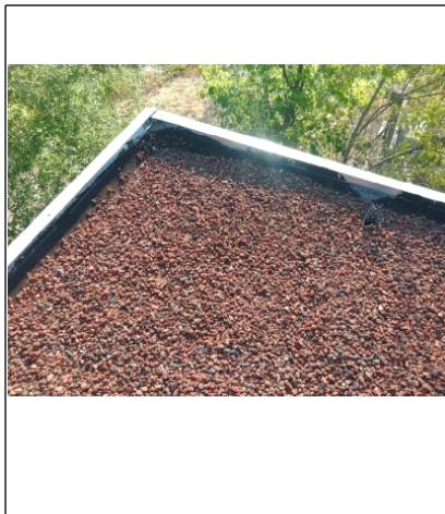
Missing flashing
