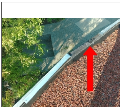
Missing flashing
