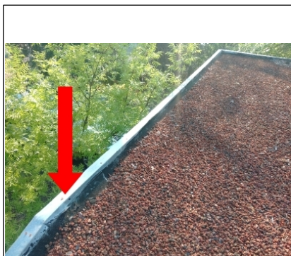
Rusted nails have allowed water to intrude through the fascia.
