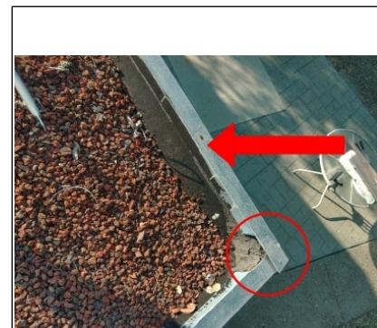
Rusted nails have allowed water to intrude through the fascia.
