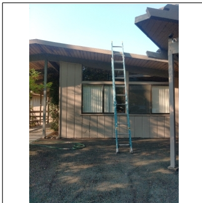
Inspected on the roof
