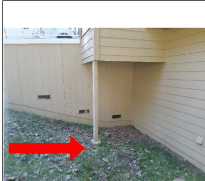
No Possible Drain Tile? recommend a diversion away from the foundation of the house
