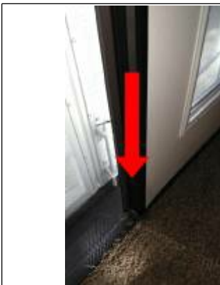
Door Stopper makes it hard to open. Possibly do to new carpet being installed.
