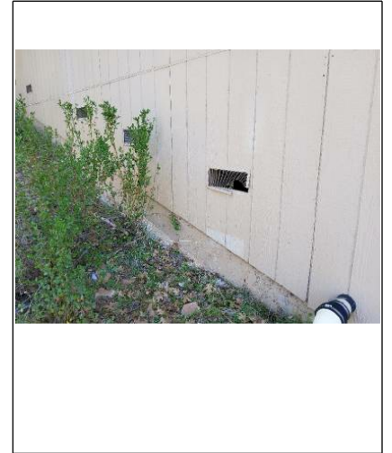
No Possible Drain Tile? recommend a diversion away from the foundation of the house
