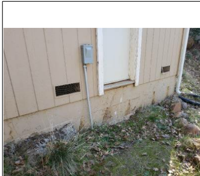
No Possible Drain Tile? recommend a diversion away from the foundation of the house
