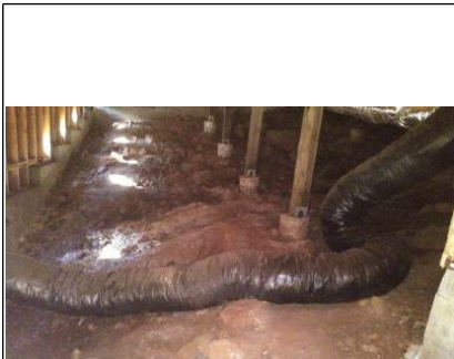
This should not be touching the ground. Duct work must always be off the ground. This is referred as handyman installing not from the builder.
