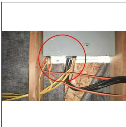
this is open light behind the panel box in the crawl space this needs to be addressed
