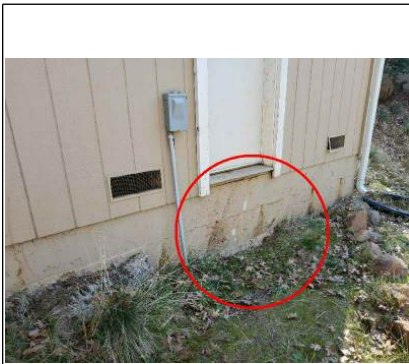
Need steps and landing pad
