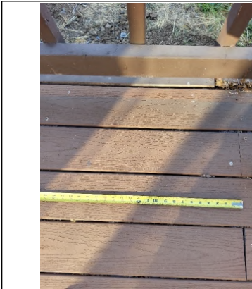
Joist layout is 2' on center.
