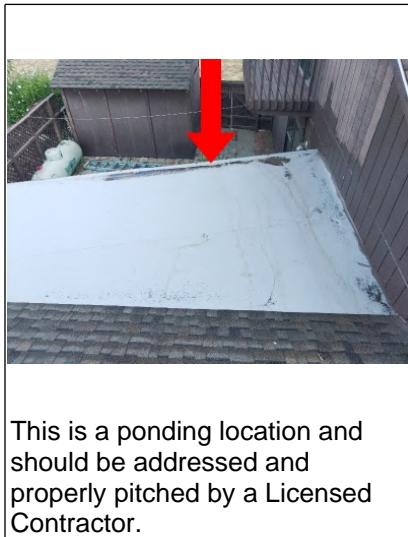
This ponding location is of concern as there is no proper pitch to the gutters at this location.
