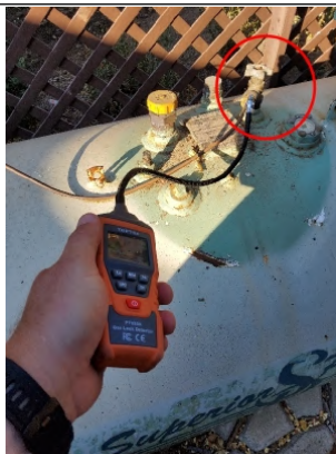
No leaks were detected on shut off valve.
