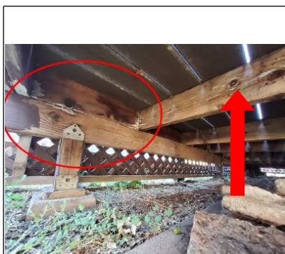
Fungus is evident on both joist and girder members. Recommend having properly treated and removed by a Licensed Pest Control Company.
