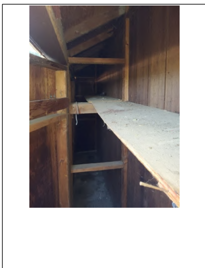
Romex electrical is exposed. This is recommended to be in conduit as the shed is still considered to be exterior.
