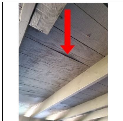
This is not of structural concern do not touch. This is T and G planking and the bottom female lip is just slightly damaged.
