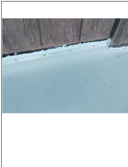
This is a ponding location and should be addressed and properly pitched by a Licensed Contractor.
