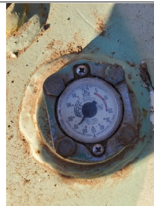
Propane tank is 70 percent full during time of inspection.
