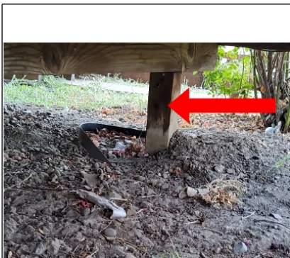
Recommend replumbing "re-leveling" all out of level posts.
