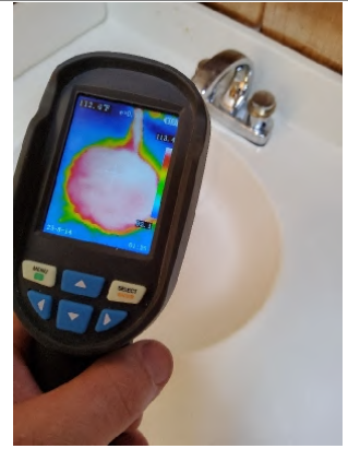
Thermal Imager shows hot water is present through shower head.
