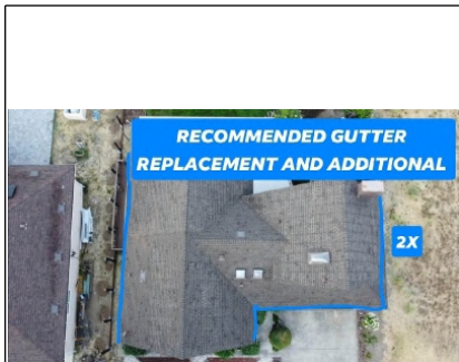
Recommended gutter replacement locations.
