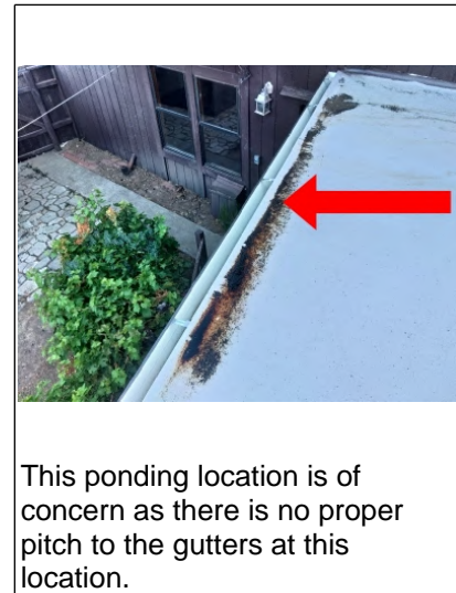
This is a ponding location and should be addressed and properly pitched by a Licensed Contractor.
