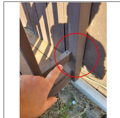
Refasten loose railing with 3" exterior screws.
