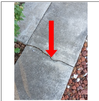
Recommend filling crack with gray polyurethane self leveling concrete crack sealant. (Comes in a caulking tube)
