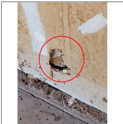
Recommend drywall patch work
