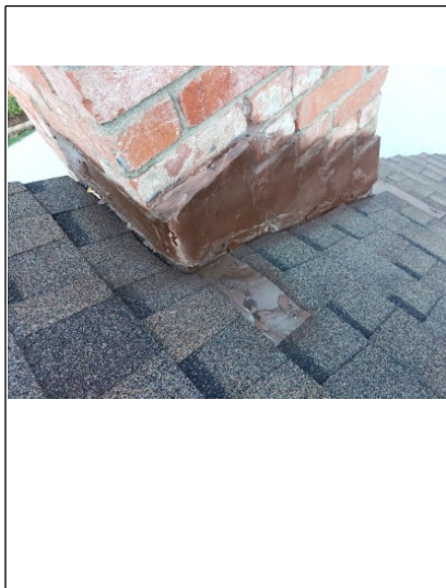
Mortar cracks are evident on chimney chase. Recommend having repaired by a Licensed Chimney Specialist.
