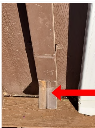
Damaged elbow
