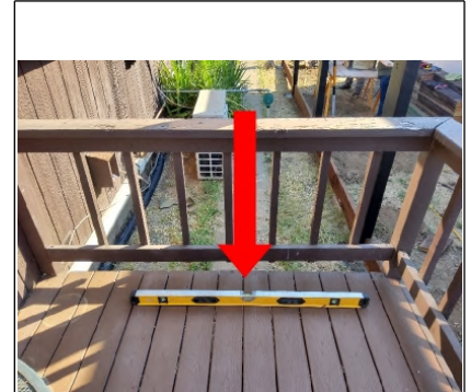
4' level is placed on top of the deck to show the deck is leaning towards the home.
