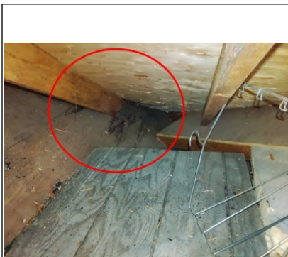
Old water stains from prior roof.
