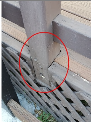
Refasten all loose posts
