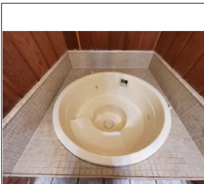
Jets were operable when testing. However, water was not tested on hot tub.
