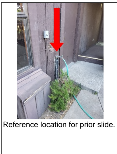
Recommend replacing corroded hose bib.
