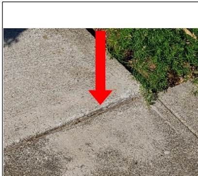
Recommend filling crack with gray polyurethane self leveling concrete crack sealant. (Comes in a caulking tube)
