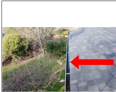
Standing water is evident. Most likely the gutter is clogged at the downspout location.
