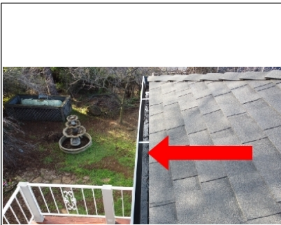
Standing water is evident. Most likely the gutter is clogged at the downspout location.
