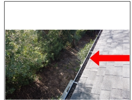
Standing water is evident. Most likely the gutter is clogged at the downspout location.
