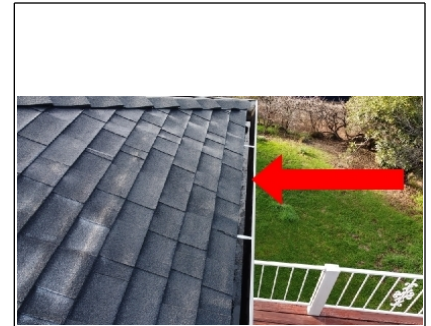
Standing water is evident. Most likely the gutter is clogged at the downspout location.
