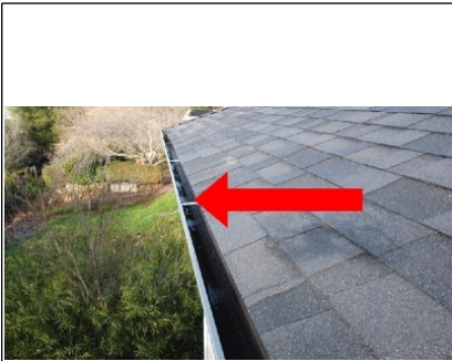
Standing water is evident. Most likely the gutter is clogged at the downspout location.
