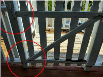
Change out hinges on gate and refasten for better closing ability.
