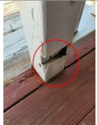
retighten 4x4 post with a lag into the rim (predrill first to avoid splitting).
