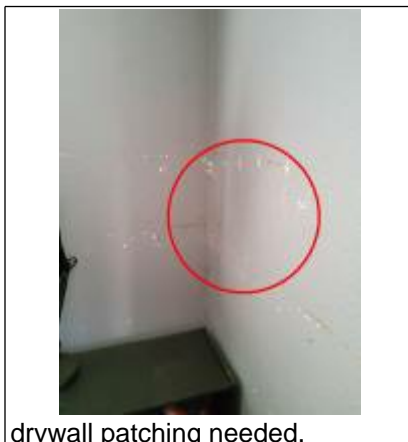
drywall patching needed.
