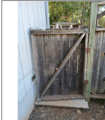
Not properly closing due hardware, installation and age.
