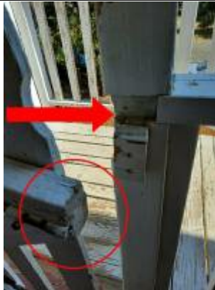
gate is sagging change out latch to a standard gate latch.
