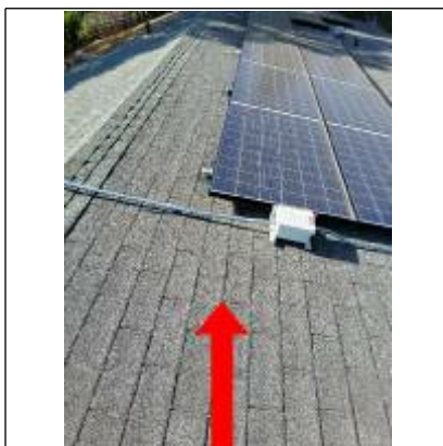
Roof needs to be replaced. In order for roofing to be replaced panels would have to be taken down. This 3 tab roofing life expectancy has been over for years.
