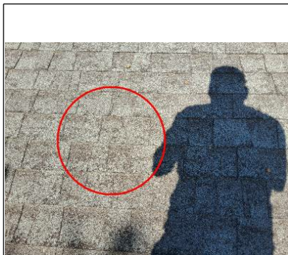
This is the sun facing dimensional roofing second layer that was installed over the 3 Tab roofing. This is the end of its life cycle and must be torn out and replaced.
