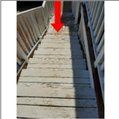
this step is a trip hazard needs to be refastened.
