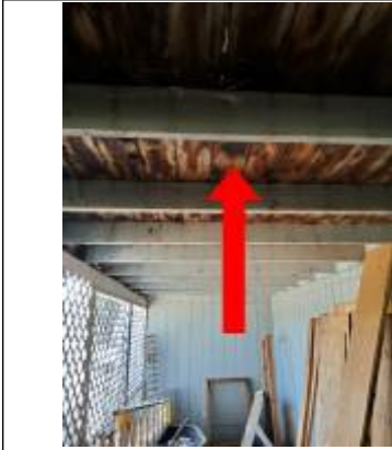
Moisture damage. However being a covered porch this is not a major concern as the deck still has kept its structural integrity.
