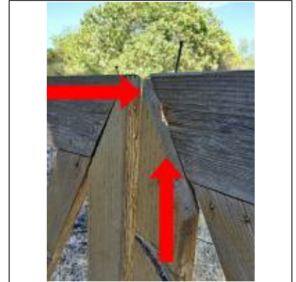
Refasten and predrill for a three inch screw from the side vertical latch board to the top horizontal board with the hinges.
