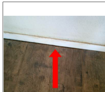
install quarterround throughout house where ending cuts of hardwood floor are exposed.
