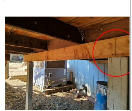
Install strong tie. (Simpson Strong-Tie 4x4)
