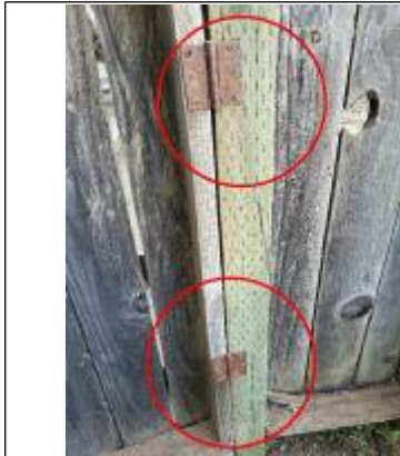
Replace hinges (Rusted))
