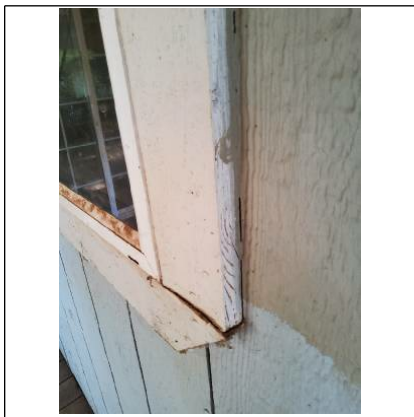
Most notable area of needed chalking
