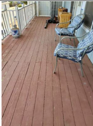
Deck could be repainted but is cosmetic
