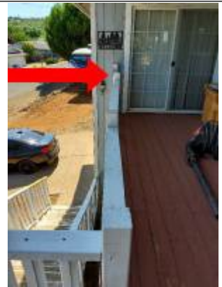
This post can be refastened with 5 inch lags going into the rim of the decking.
