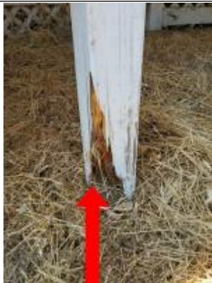
use a jack and replace 4x4 post with pressure treated or DF on top of either cinderblock or post block
