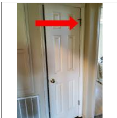
Run 3 inch screw in hinge to ease operation.
