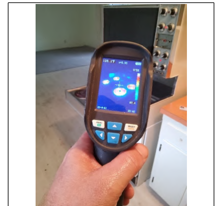
Thermal Imager shows all burners show proper operation.
