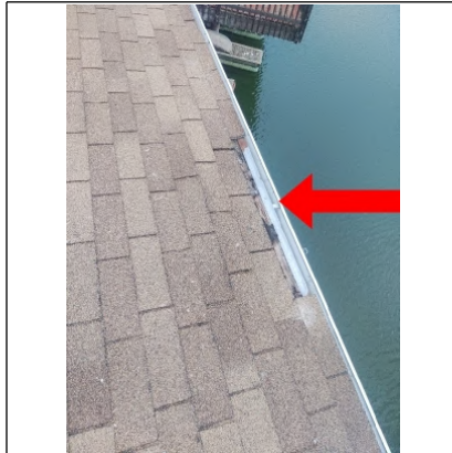
Missing shingle location
