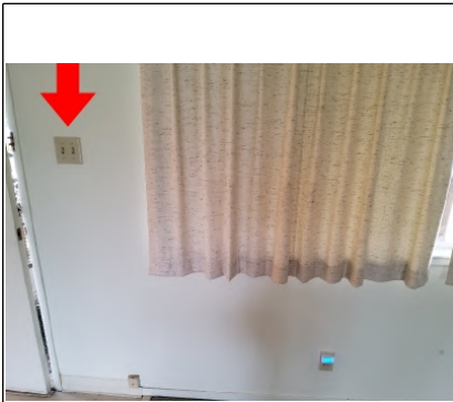
Switch location for outlet.
