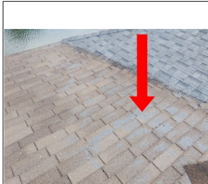
Missing shingle location
