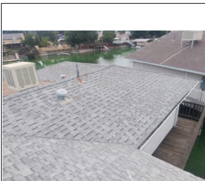
30-Year Asphalt Dimensional Shingle
