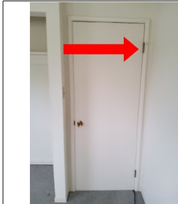
Recommend tightening door jamb to properly latch door. Take off the middle screw on top of the hinge pre-drill with a drill bit then get a 3 screw with a large enough head to flush the hinge. This will tighten the jamb to the trimmer allowing the door to close with ease. Recommend taking the existing screw out to match heads with the new replacing screw.
