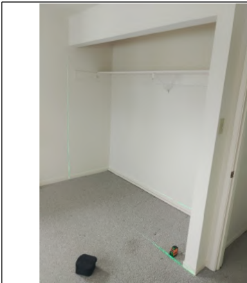
Laser level shows walls are plumb.
