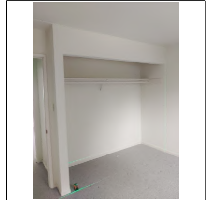
Laser level shows walls are plumb.
