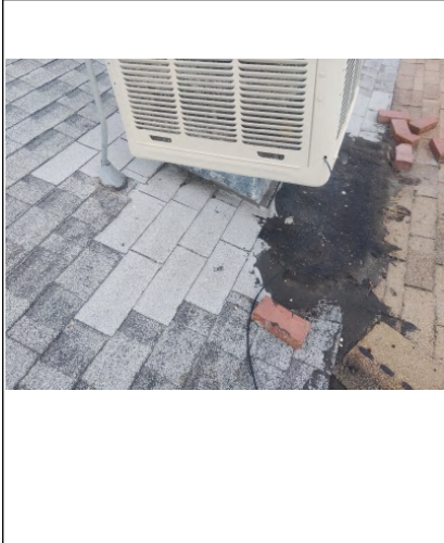
Recommend having a 3/4" PVC drain line installed on swamp cooler.
