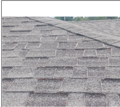
Reference section #2 with regards to worst conditioned shingle location. (Refer to diagram for locations)
