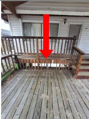
Water shut off location
