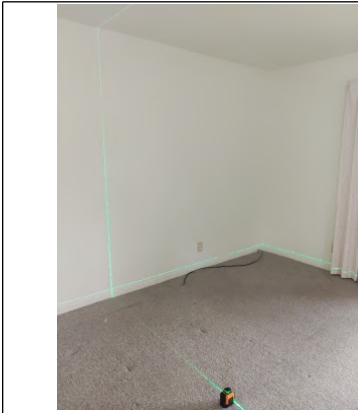
Laser level shows walls are plumb and floor is level.
