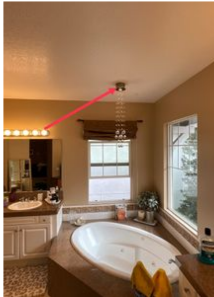
EXHIBIT 410.1 Luminaires, lighting track, and suspended (paddle) fan located near a bathtub.
