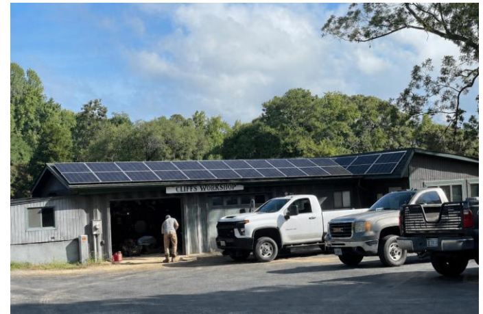
Building with solar panels
