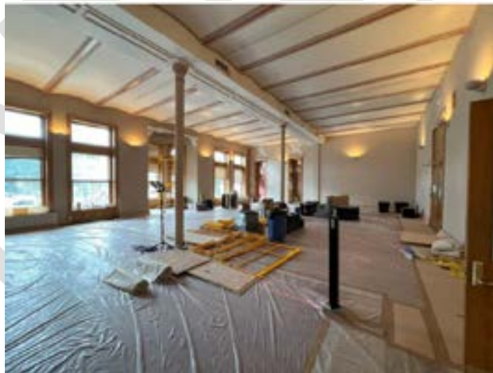
Figure 92: Salt Lake County Building Earthquake Repair Project 110
