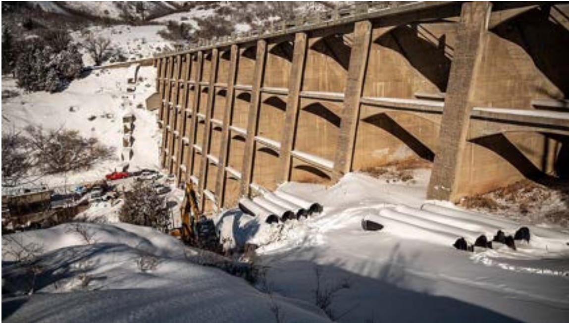
Figure 57: Mountain Dell Dam 63
