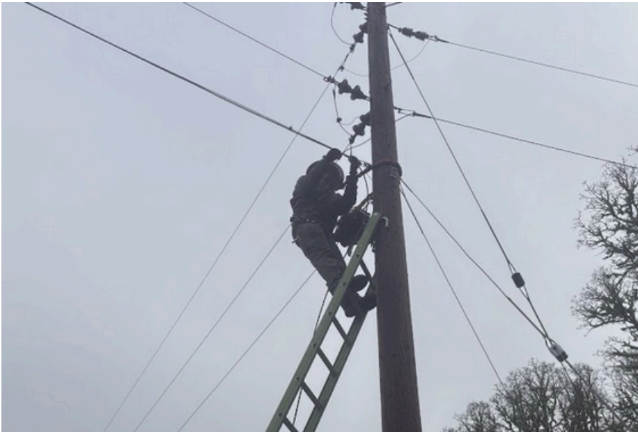
Outside Plant Team Member Oliver, going where the bucket trucks can't
