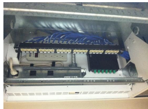
FSR CB-224 with fiber, copper and AC connectivity
