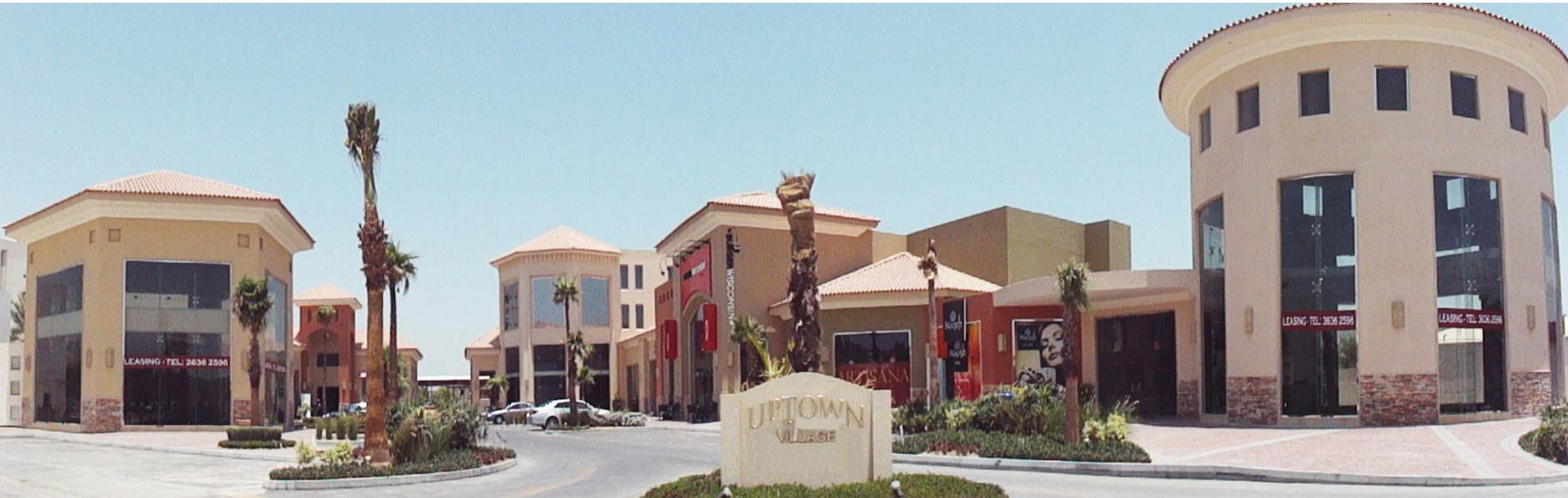
This chic shopping development utilized Cellate Large panel technology throughout. The buildings to the top right were geometrically complex with large unsupported flooring spanning up to 10 meters across. All Panels were cast on site to the back of the development which became the car park after building completion. This project was completed ahead of the original program in 4 months.
