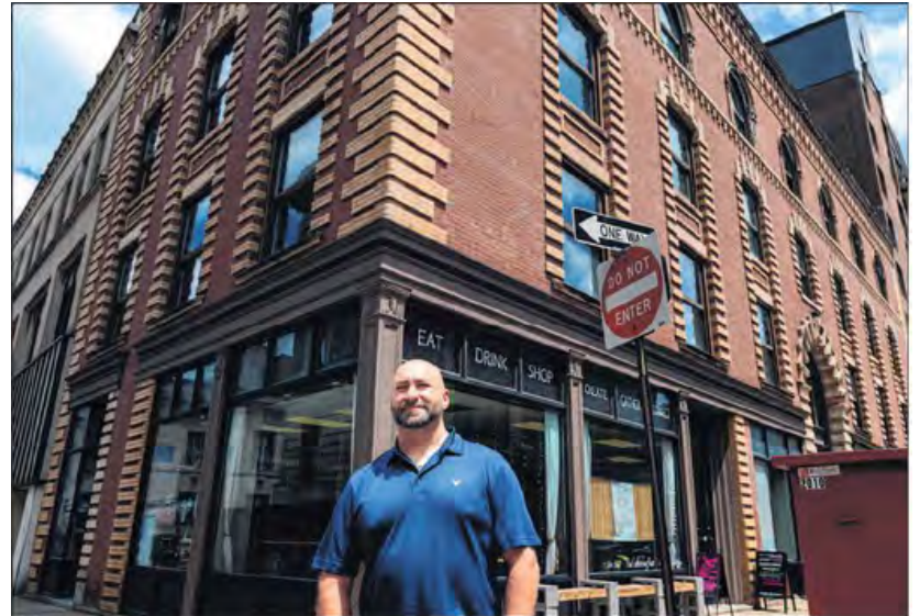
Kirk Mariolis of M4 Investment Group LLC., talks about his family's investments in eight buildings in downtown Waterbury including the building at the corner of Center Street and Leavenworth.
