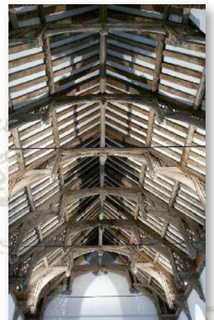
The hammer-beam roof of St Mary the Virgin church.
