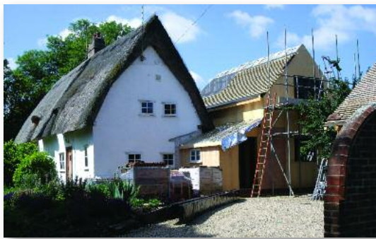
Extension awaiting cladding with traditional tile and render.
