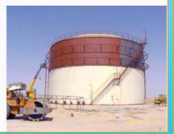
\* THE DESIGN OF THE TANK IS BASED ON THE AMERICAN SYSTEM **FOR** THE (API DESIGN OF VERTICAL **TANKS** STANDARD 650 \ 620). THE ENGINEERING DESIGN IS DONE USING THE LATEST SPECIALIZED PROGRAMS BASED SUCH **AS** INTERGRAPH TANK. THE **ENGINEERING STUDY IS CARRIED OUT BY** A SPECIALIZED ENGINEERING TEAM.
