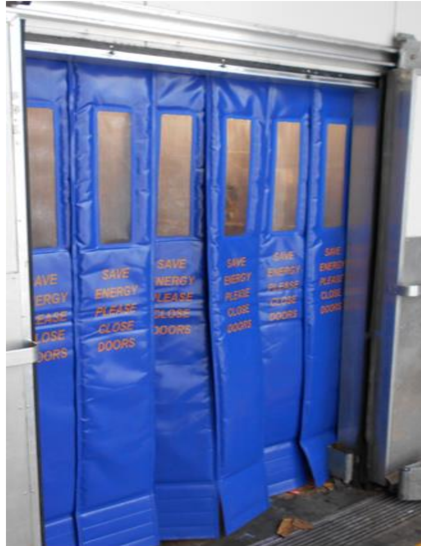
Post Installation Cool Room Door – External View
