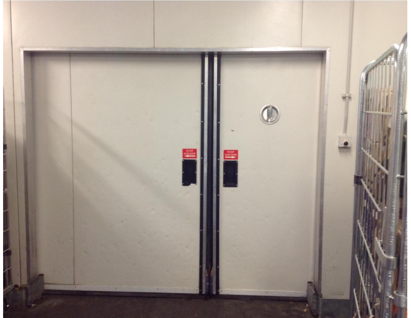
Pre Installation Cool Room Door – Internal View
