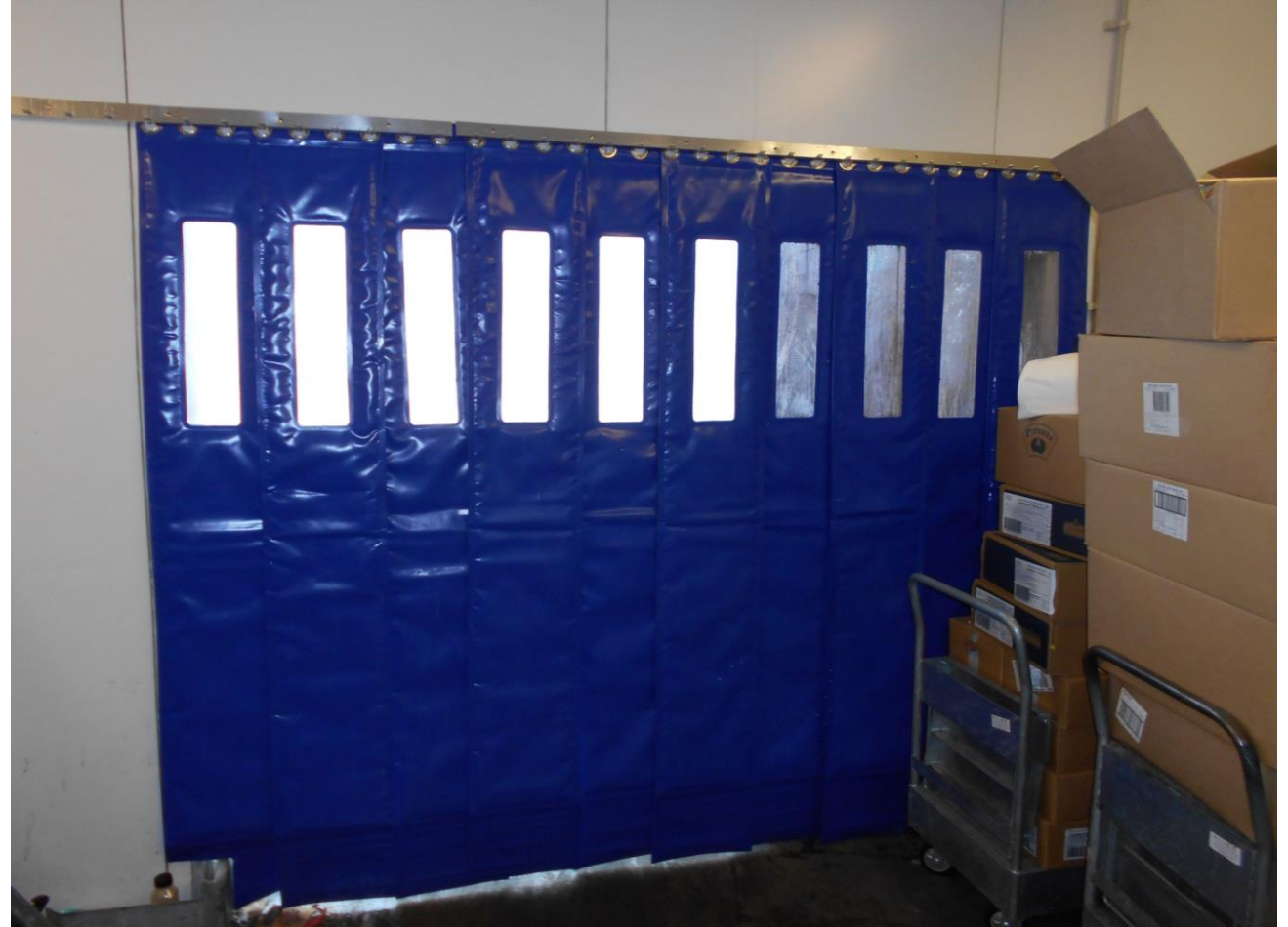
Post Installation Cool Room Door – Internal View
