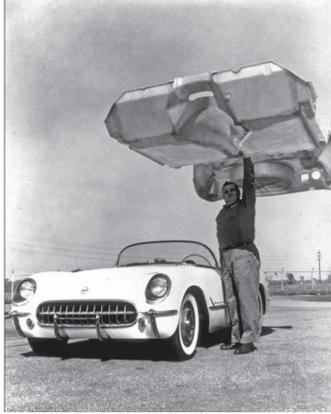
Corvette's use of advance materials began in 1953, when the first Corvettes were produced with all-fiberglass bodies. Every Corvette since has featured a composite-material body. Over the years the make up of the bodies on the Corvette has changes dramatically as technology has advanced,
