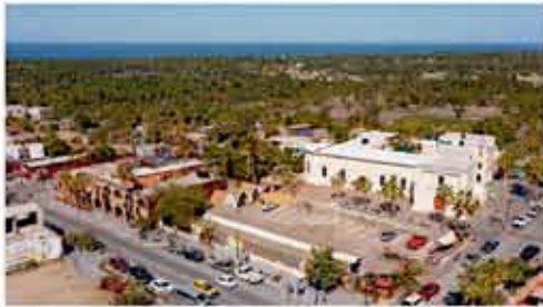
Hotel California Parking Lot 1,459 m 2 prime location
